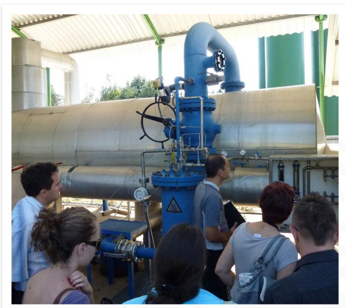
Production well of a doublet in a carbonate reservoir in Bad Blumau, Austria, with a degassing unit
