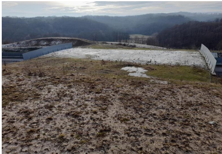
Fig 4. The surface of the green-bridge near Bastea is not attractive for wildlife as the land is eroded by grazing © Zarand
