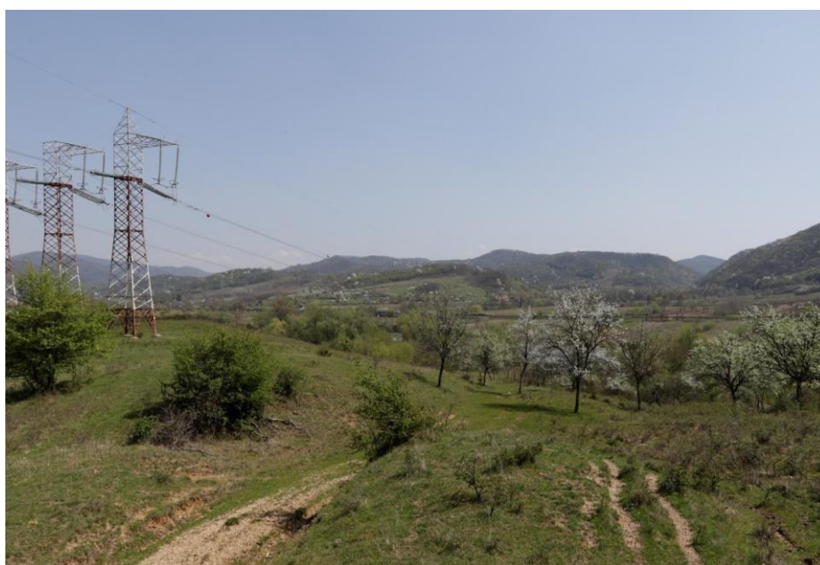
Fig 3. The land-use on top of the Pojoga tunnels of the Paulis –Deva upgraded railway is complex; thus, adequate management regulations are mandatory in order to ensure functional connectivity © Zarand
