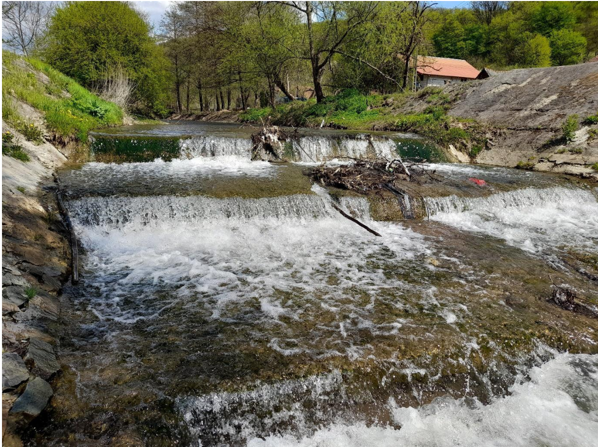
Fig 9. Example of a barrier for local fish species on one of the Mures tributaries © Zarand
