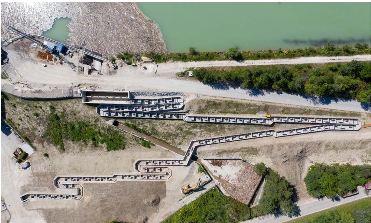
Figure 10 Example of a fishway built in Austria, to overcome a barrier of 26 metres (© VERBUND AG)
