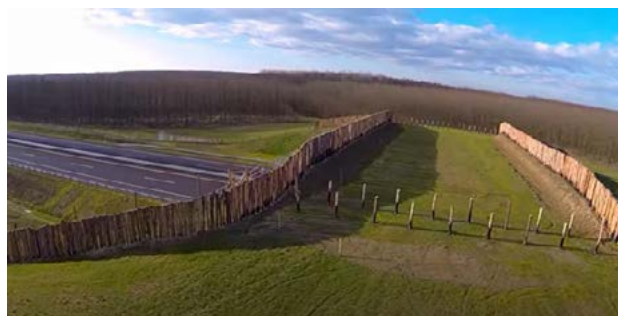
Existing wildlife overpass on M3 motorway in Hungary (Source: https://magyarepitok.hu/vasarosnamenyig-er-az-m3 )
