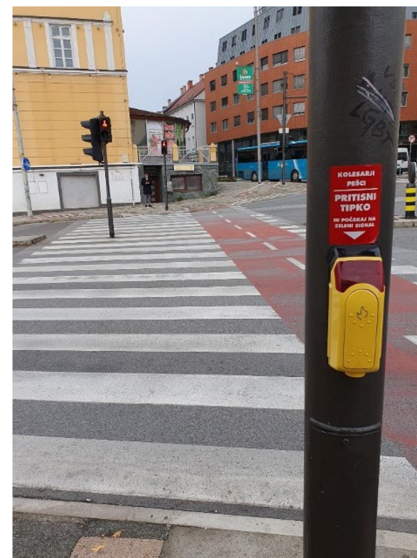
Acoustic signals for traffic lights at two pedestrian crossings at the northern intersection of the main bus station
