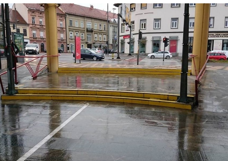
Contrasting markings – main entrance stairs
