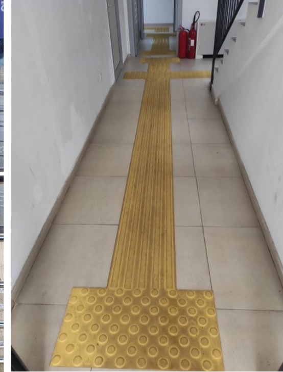
Entrance to terminal and indoor TWSIs guiding to sanitary facilities
