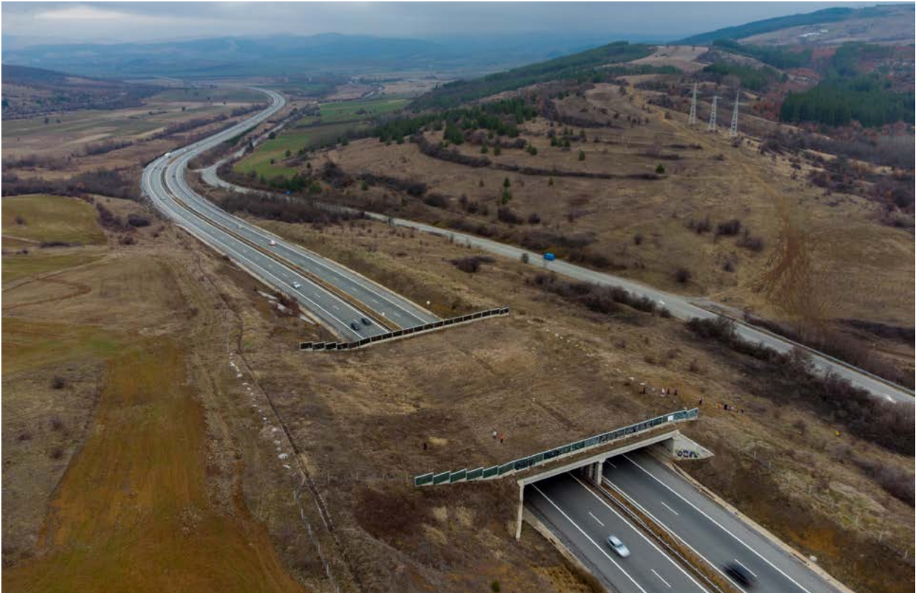
Fig 16. A bear overpass at Struma Motorway Section 1 viewed from above. Ploughing of the adjacent arable land on the left western side and the presence of the 1st class road as well as the lack of guiding vegetation on the right eastern side of the overpass further reduce the permeability of the transport infrastructure (© BBF).
