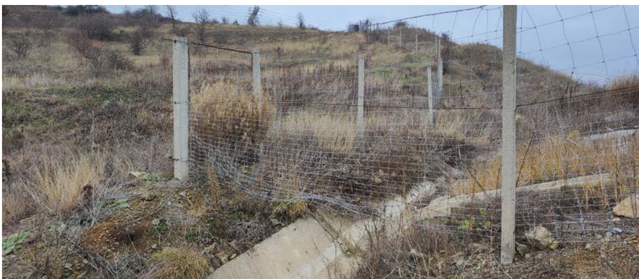
Fig 18. The existing fence is not bear-proof and not well fixed to the background, and not maintained regularly (© BBF).
