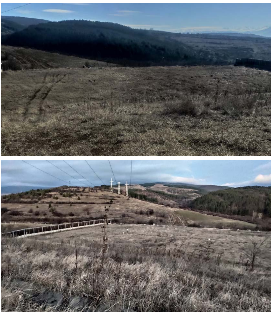
Fig 9. An overpass for bears at Struma Motorway Section 1 with missing micro-habitats and hiding structures. (© BBF).
