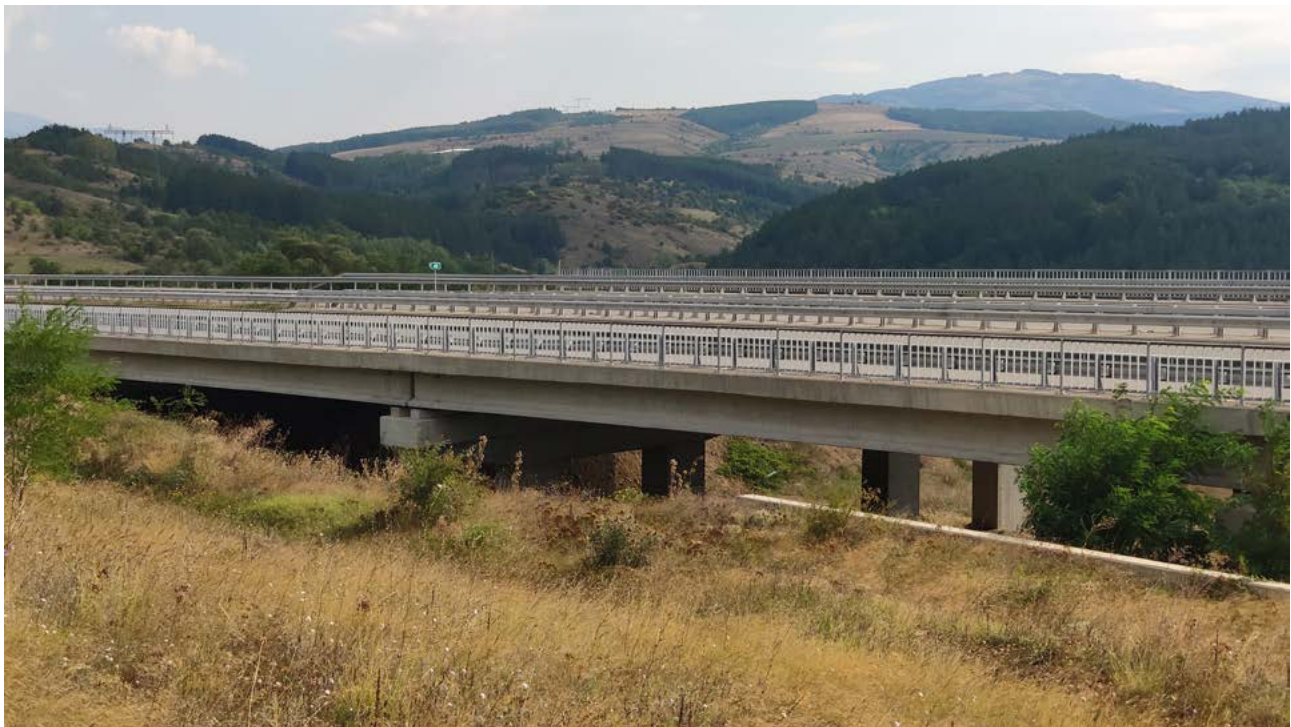
Fig 10. A low non-specialized viaduct at Struma Motorway Section at 1 km 314+400, 42°22'23.87", 23° 6'42.18" serves as an effective wildlife crossing, but needs some improvements. (© BBF).
