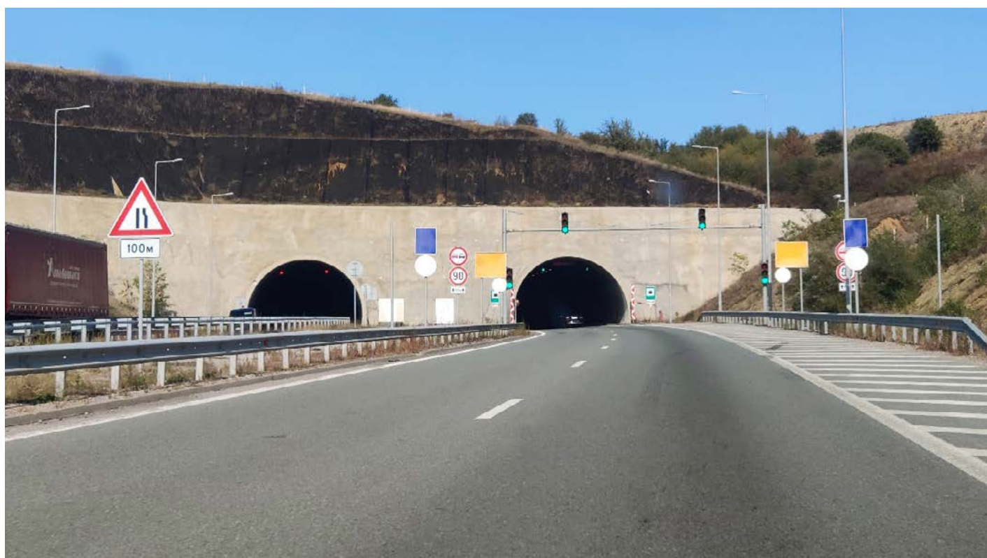
Fig 7. The tunnel at the Struma Motorway Section 2 is functioning as a non-specific ecoduct from km 324+460 up to km 324+840, 42°17'13.33" 23° 5'11.37"
