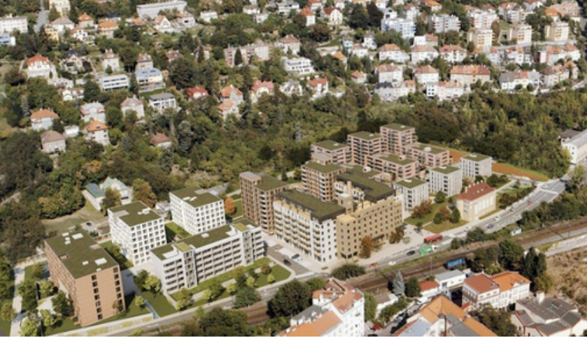
"Odkolek area after revitalization" (c) City of Prague
