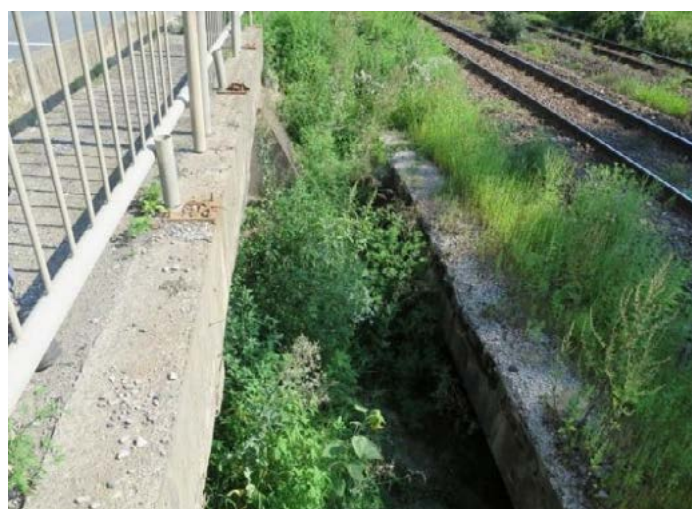
Figure 13 Example of a blocked small bridge/culvert on the old railway – Km 566+100 (© Zarand)
