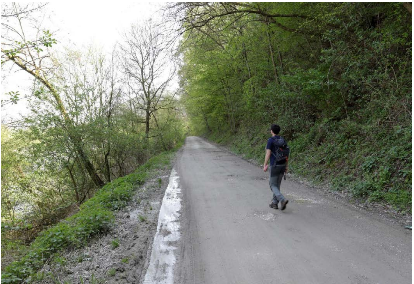
Figure 11 Original state of the county road DJ 707A., currently having steep slopes. Any increase in the barrier effect during the upgrade may make the tunnel area non-functional (© Zarand)
