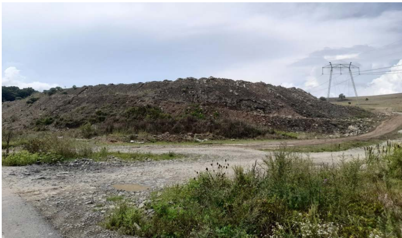
Figure 24 Damping site created near a green-bridge (© Zarand)
