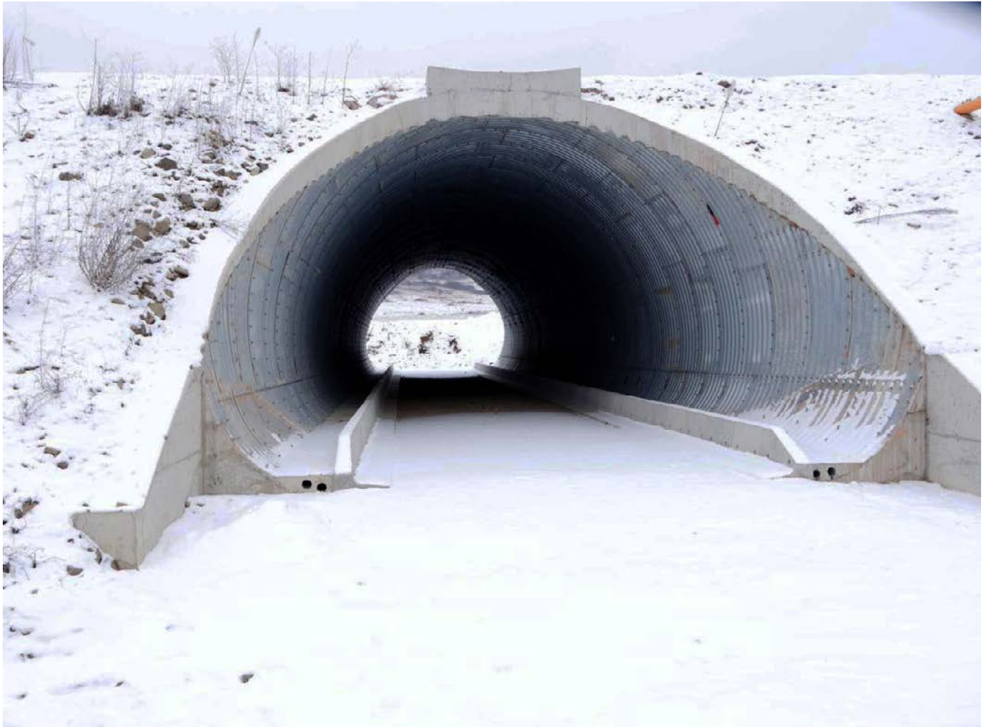
Figure 4 A large rectangular passage included in the initial technical plan was changed into a semi-circular, reduced-in-size object, diminishing drastically its potential use for wildlife. (© Zarand)
