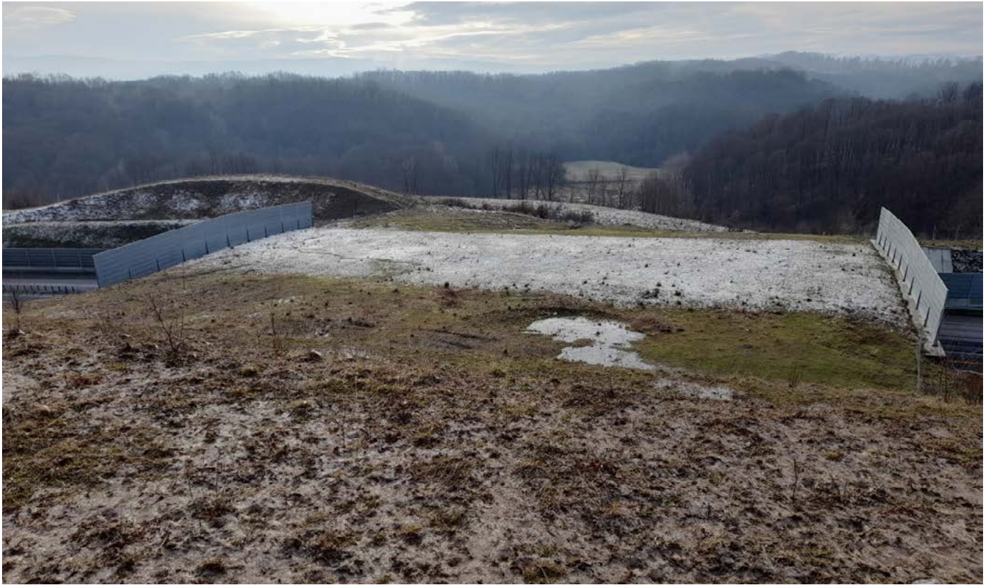
Figure 8 The surface of the green-bridge near Bastea is not attractive for wildlife as the land is eroded by grazing (© Zarand)
