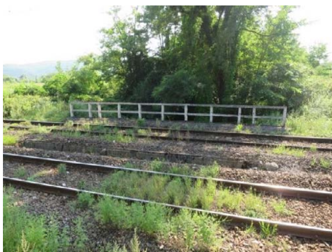
Figure 13 Example of a blocked small bridge/culvert on the old railway – Km 566+100 (© Zarand)
