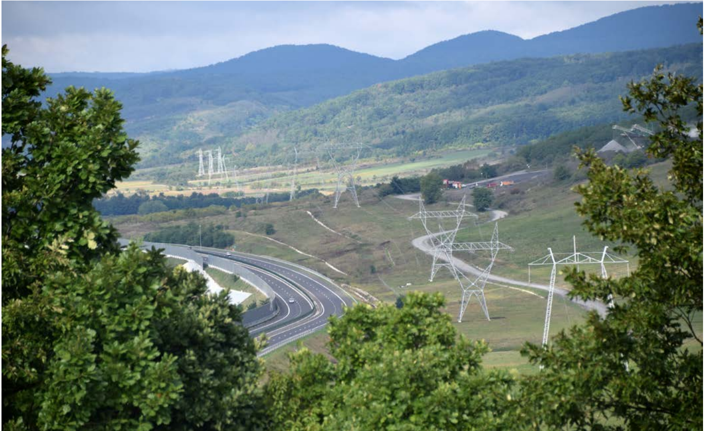
Figure 19 Power lines parallel with the A1 motorway in the Mures Valley (© Lazaros Georgiadis)
