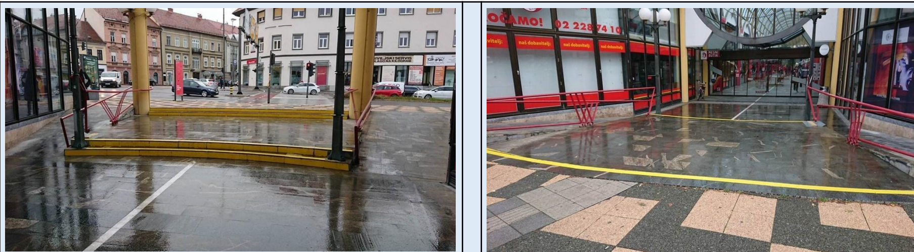
Picture 2: Contrasting strip – main entrance stairs
