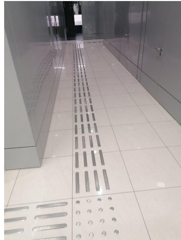
Picture 3. TWS's basement – terminal building
