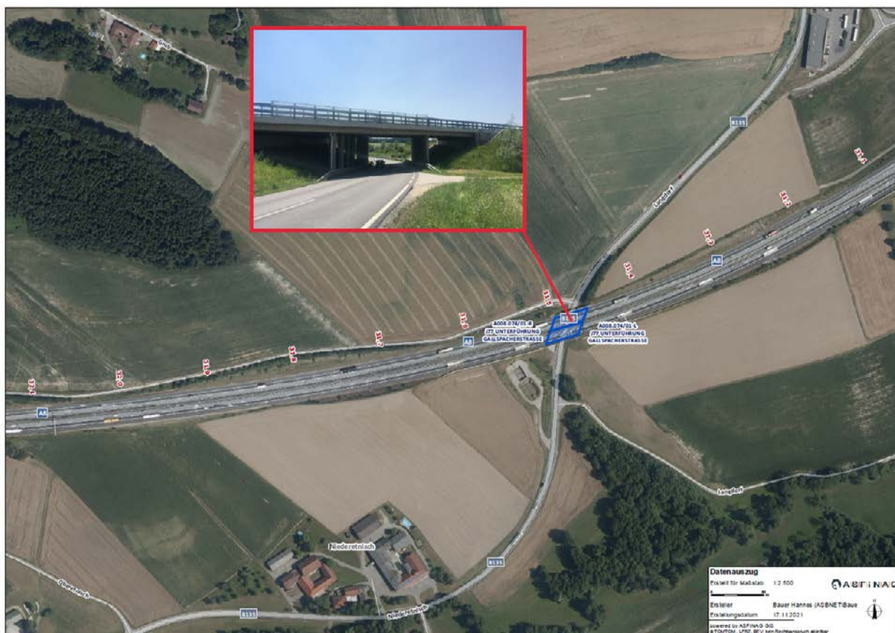
Figure 8 Western underpass near Aistersheim ©ASFINAG
