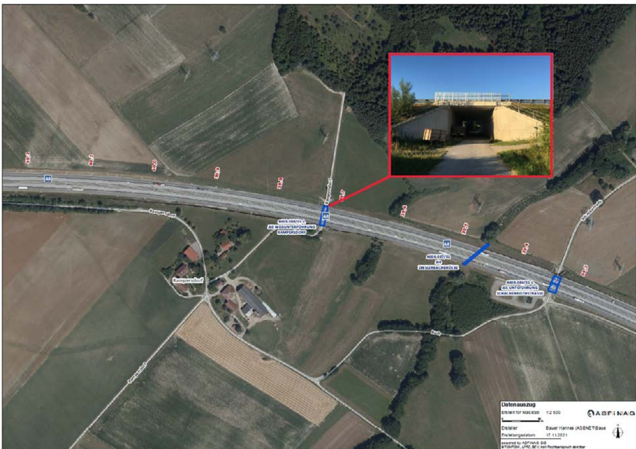
Figure 6 Underpass near Rampersdorf ©ASFINAG
