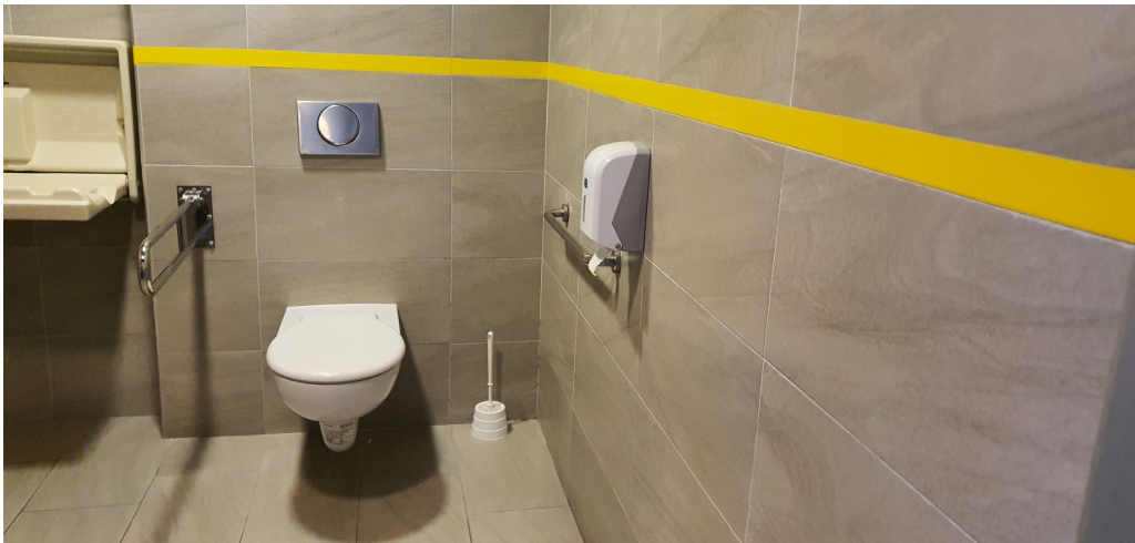
Figure 5. Contrasting tape at accessible toilets
