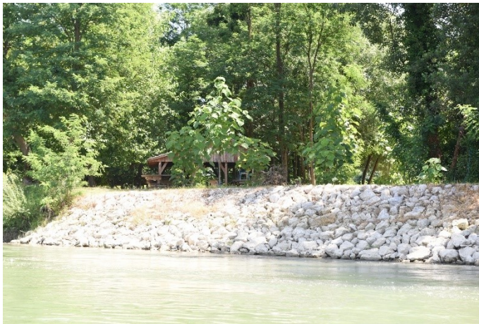
Figure 26: Rip-rap on the river bank of the Drava River and invasive species Paulownia tomentosa in Croatia in 2021. Photo: Darko Grlica.
