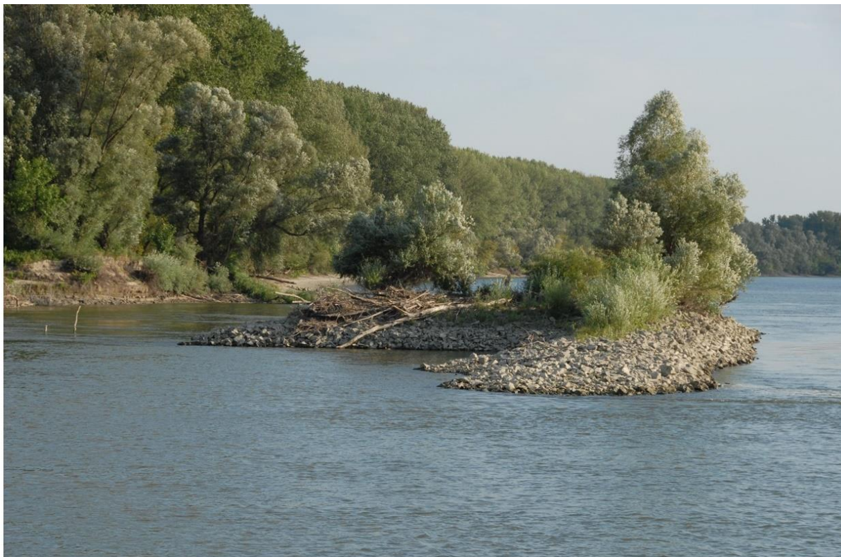
Figure 8: On the Danube T-groynes (in this case disconnected from bank) can be find in larger numbers end size to stabilize the fairway. © Credit: Wolfgang Kraier.
