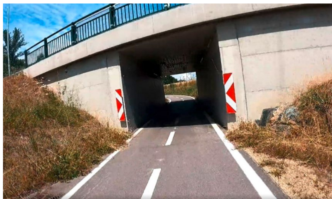
Figure 33: Underpass in Tulln/Austria
