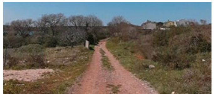
Figure 14: Presence of unpaved / gravel road at EuroVelo 8 in Croatia
