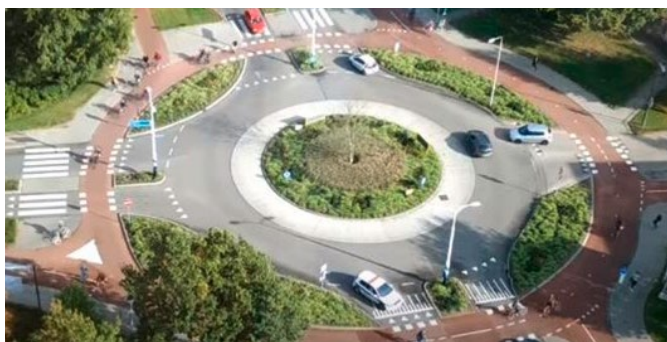
Figure 32: Segregation of two-way cycling facility and motor vehicle traffic on a roundabout in the Netherlands
