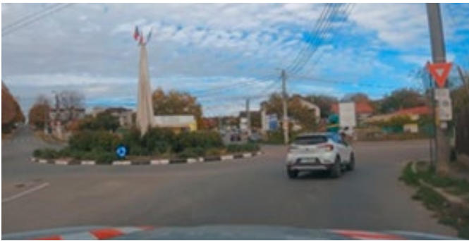
Figure 11: This roundabout in Tulcea, Romania, is lacking any markings (central, cycle path, lanes) and makes it very difficult to navigate by cyclists and drivers together.
