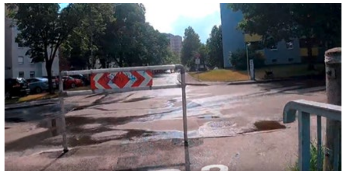
Figure 18: Railing as obstacle at EuroVelo 14 in Austria
