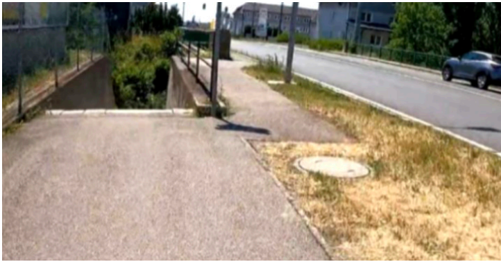
Poorly accessible underpass due to stairs at EuroVelo 9 in Austria [13]
