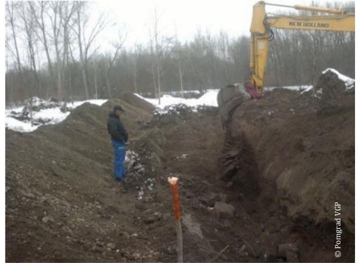
Apače secondary channel excavation
