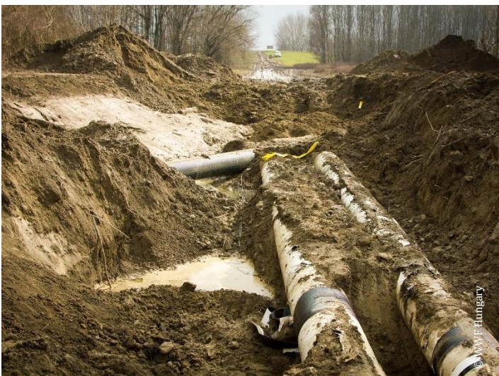
Relocation of the water pipes
