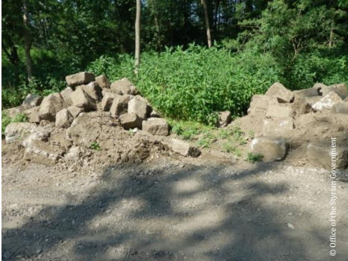
Removing of the bank protection 2012
