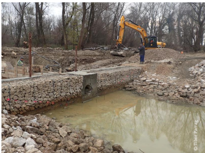
The site of the construction
