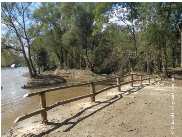
Widening of the Mura riverbed 2012, view upstream
