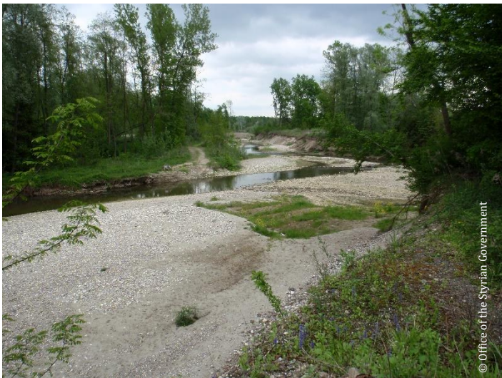
Prolongation of tributary „Saßbach“ in the new side channel, May 2010
