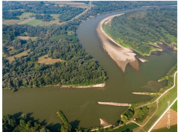
Restoration site “Novačka”: Site overview – Initial channel planned in order to ease the bottleneck and pressure on the left dike
