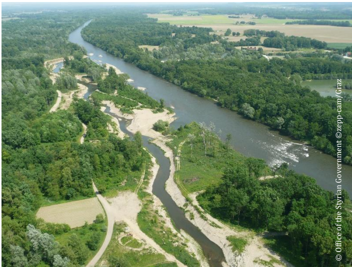
Development of the new side channel , May 2008,
