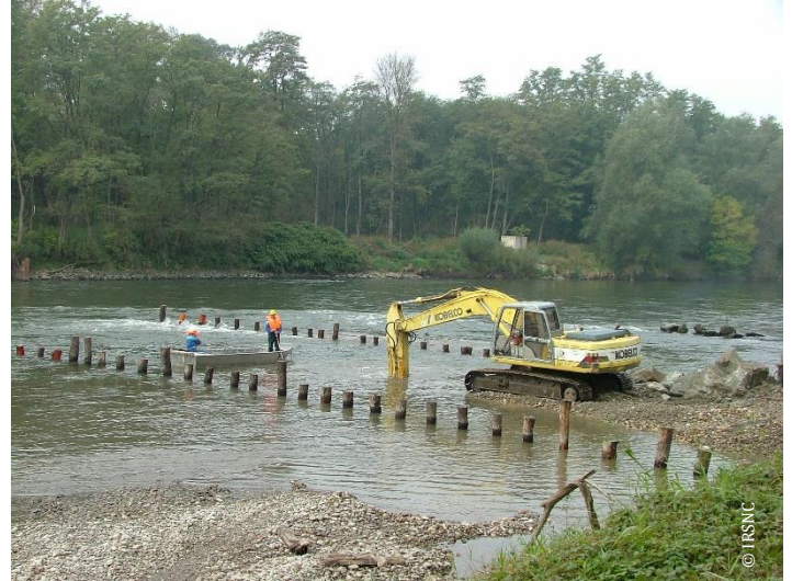
Building of the river ramp on Mura
