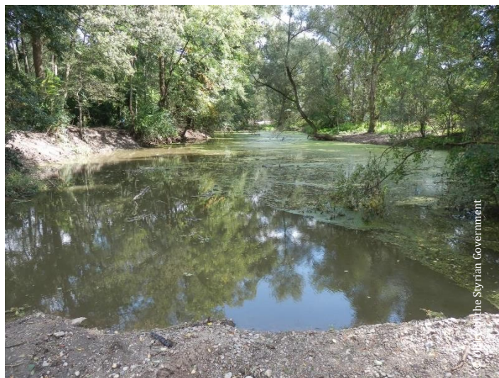
Floodplain water body during implementation 2012, view upstream
