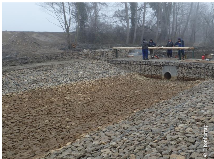
The site of the construction
