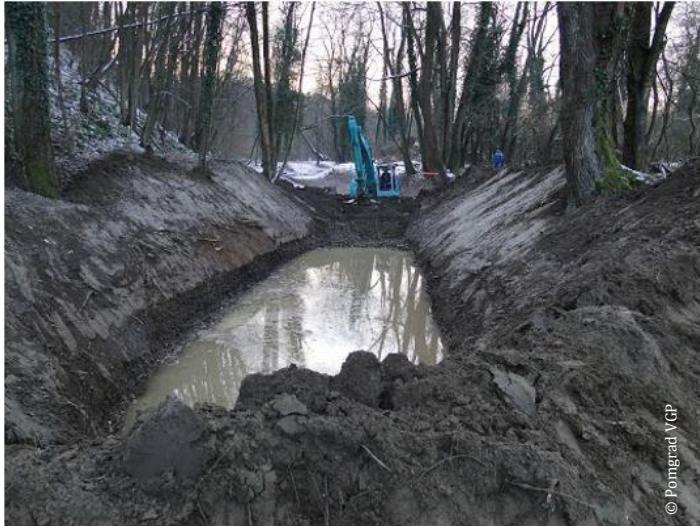
Alter Graba secondary channel excavation
