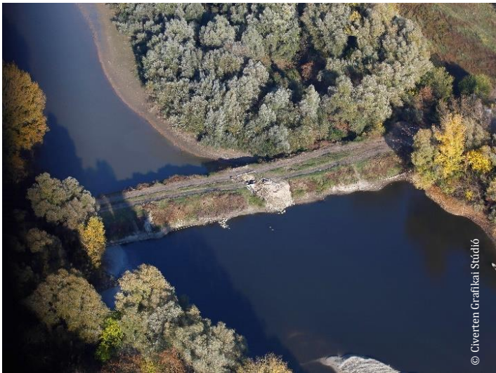
Rockfill dam which blocks the side branch before the restoration, 2012
