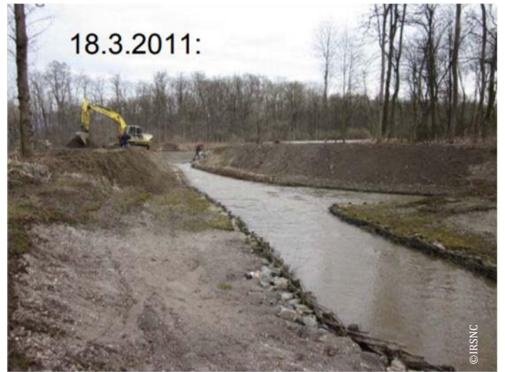
Bank opening and the secondary channel connection to the river at Besnica 2010/2011
