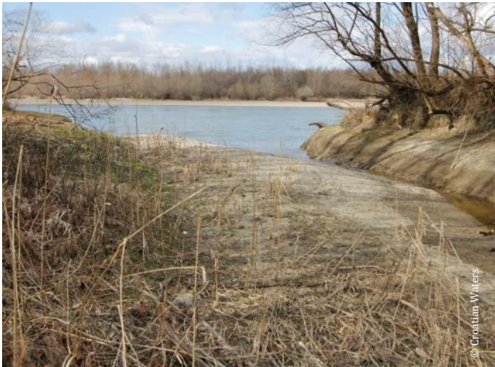
Restoration site “Donja Dubrava – Legrad”: Side channel entrance area, gradual sedimentation noticeable
