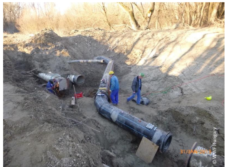
New water pipes
