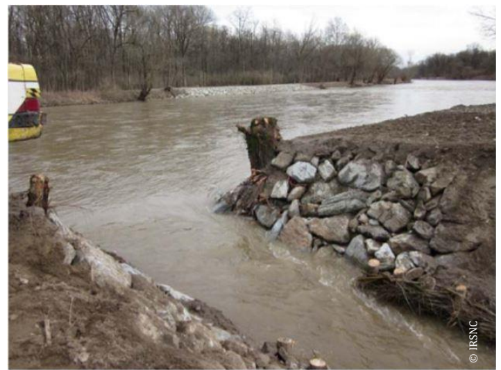
Bank opening and the secondary channel connection to the river at Bunčani
