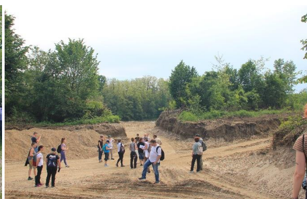
Figure 4: Construction works in Gosdorf © IRSNC
