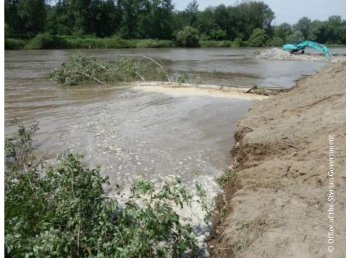
Fixing wooden structures in the new riverbank 2012, view upstream
