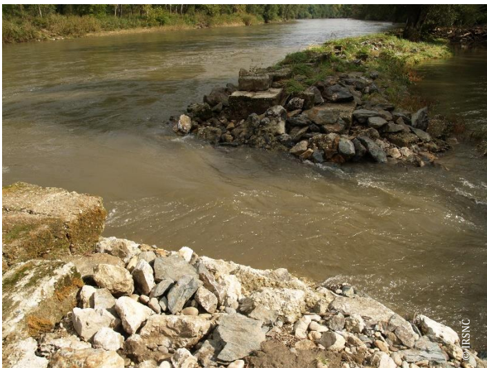
Restored inflow into the secondary channel
