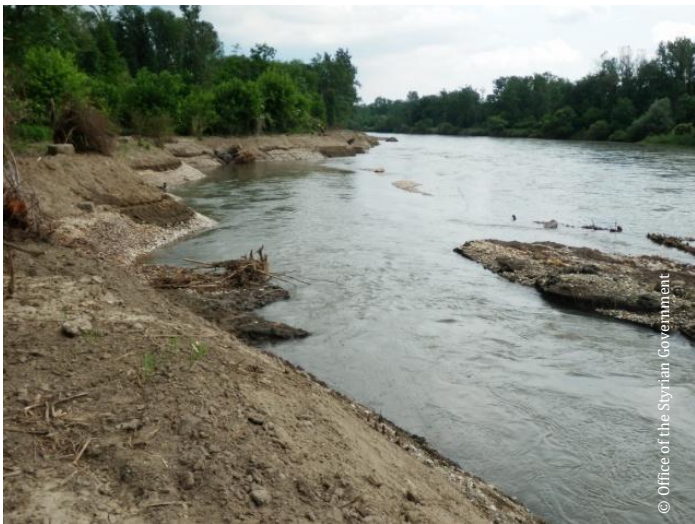
New riverbank formed by machines, May 2012, view downstream
