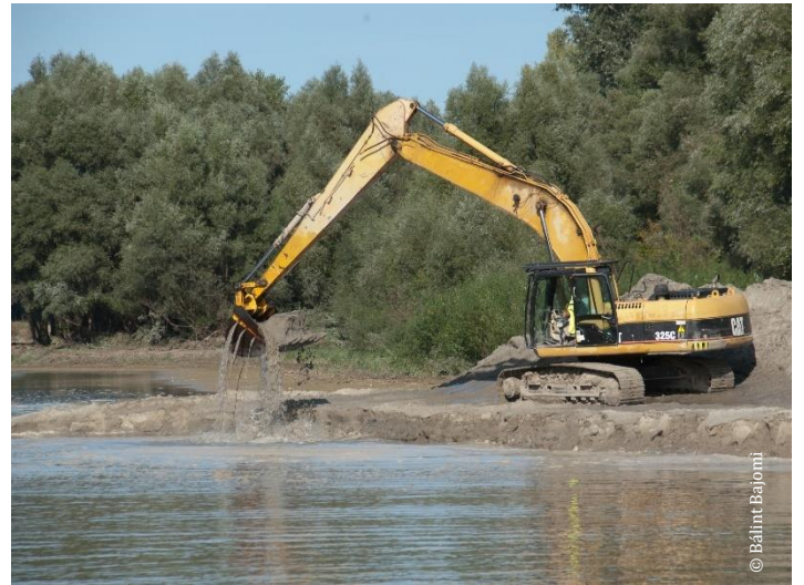
Channel dredging in the side branch
