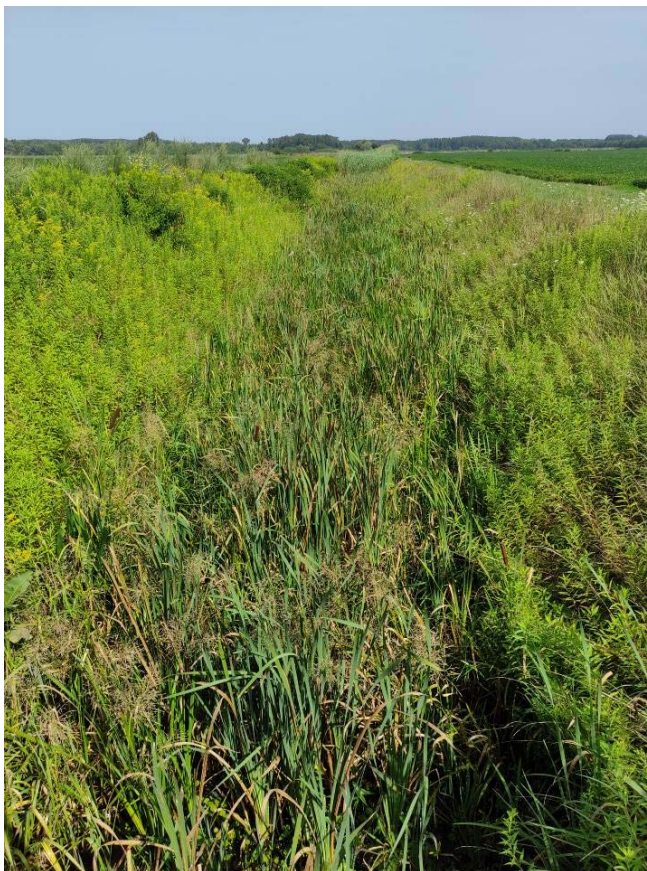
Figure 3. Labudnjača drainage channe
