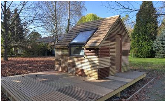
Picture 3: Testing field at the model facility
