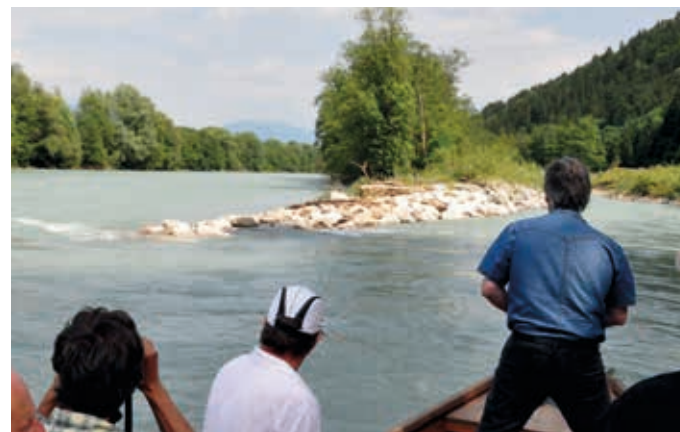
Fig. 90: Curved groyne dividing the water flow between river and initial channel (Upper Drava, Austria).
