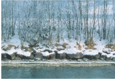
Fig. 11: Riverbed incision can have serious and costly consequences, such as undermined bank protection or unstable bridge foundations.
