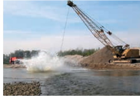
Fig. 12: Large quantities of bedload (about 200.000 t per year) are still irretrievably lost from the river system through dredging.
