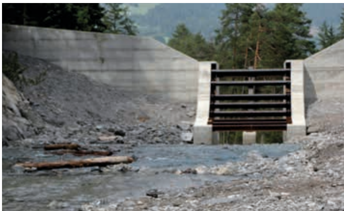
Fig. 77: New opened bedload retention dam on Feistrizbach (Upper Drava, Austria). The old dam was removed, the retention area emptied.
