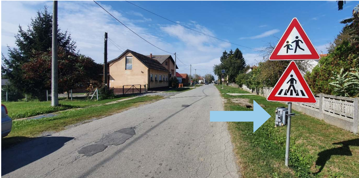
Figure 9 Automatic traffic counters installation
