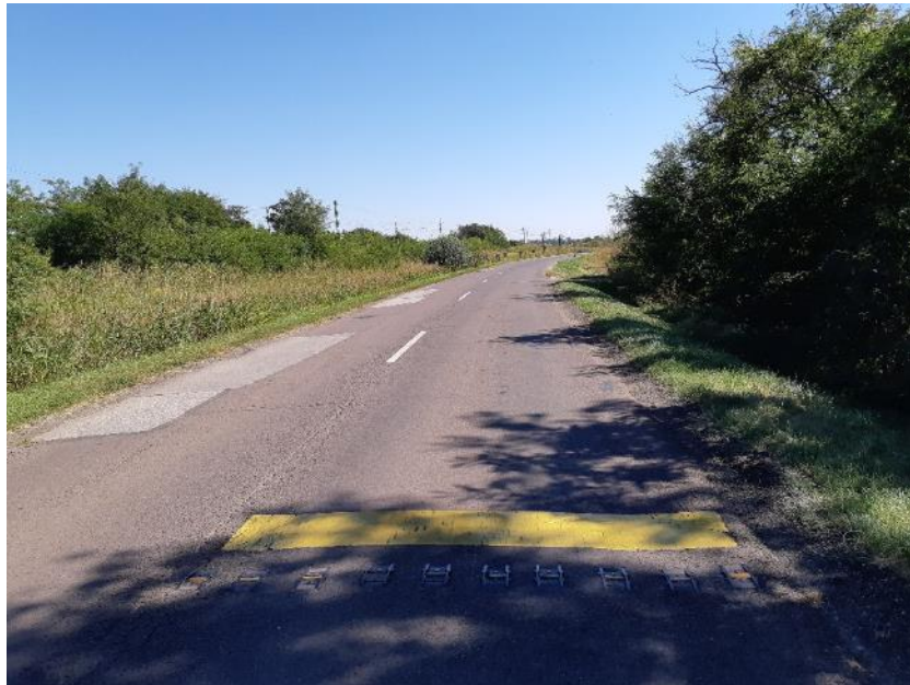
Figure 24: Area of Pilot Action 1 near Cegléd, on road 40 – 2. direction
