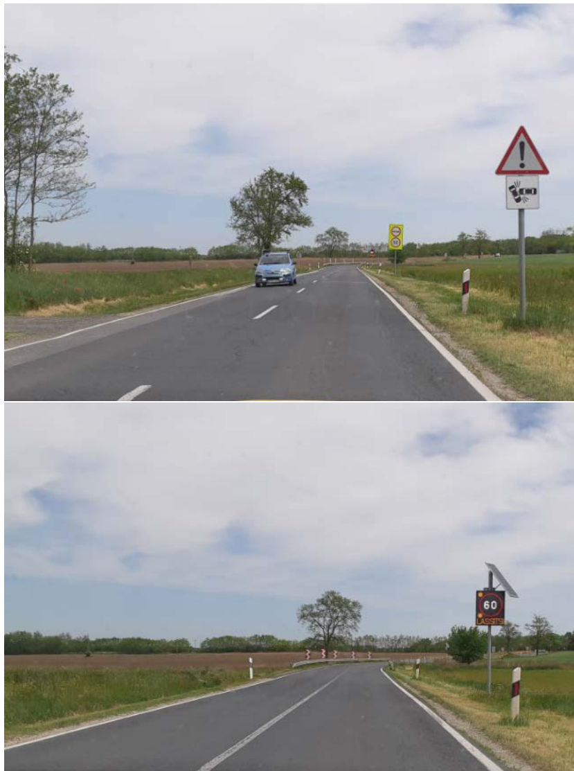
Figure 9: Measured section on road 83 with vehicle activated 60 km/h speed limit display
