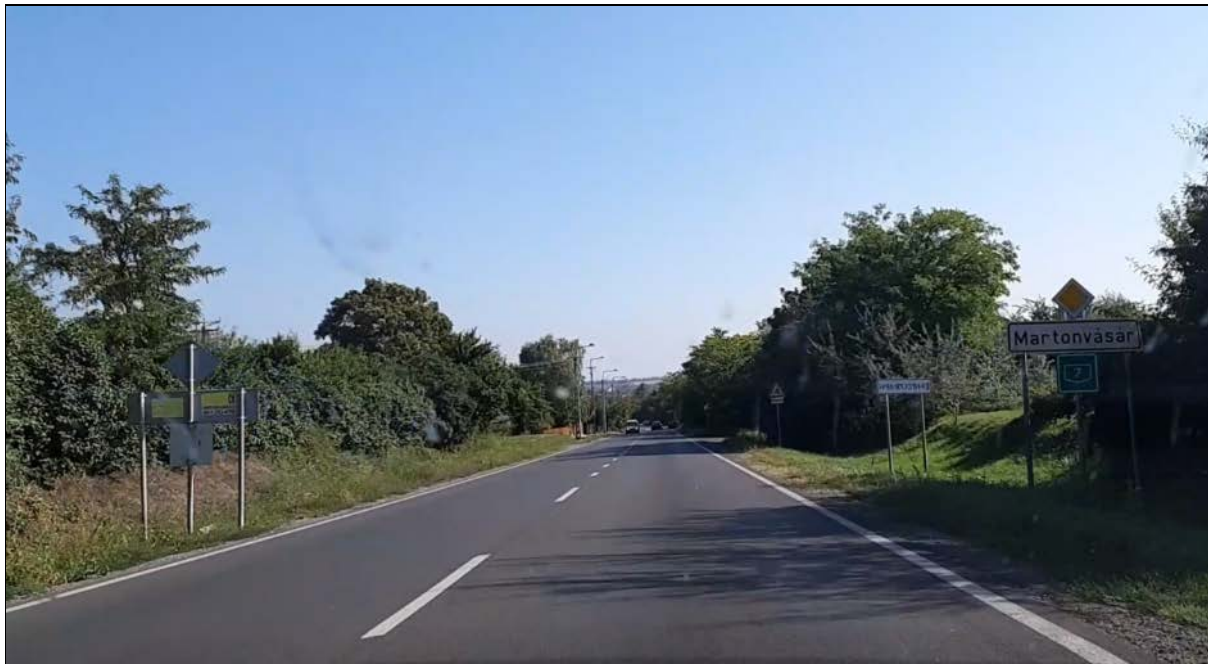
SRS – BEFORE COUNTERMEASURES IMPLEMENTATION
