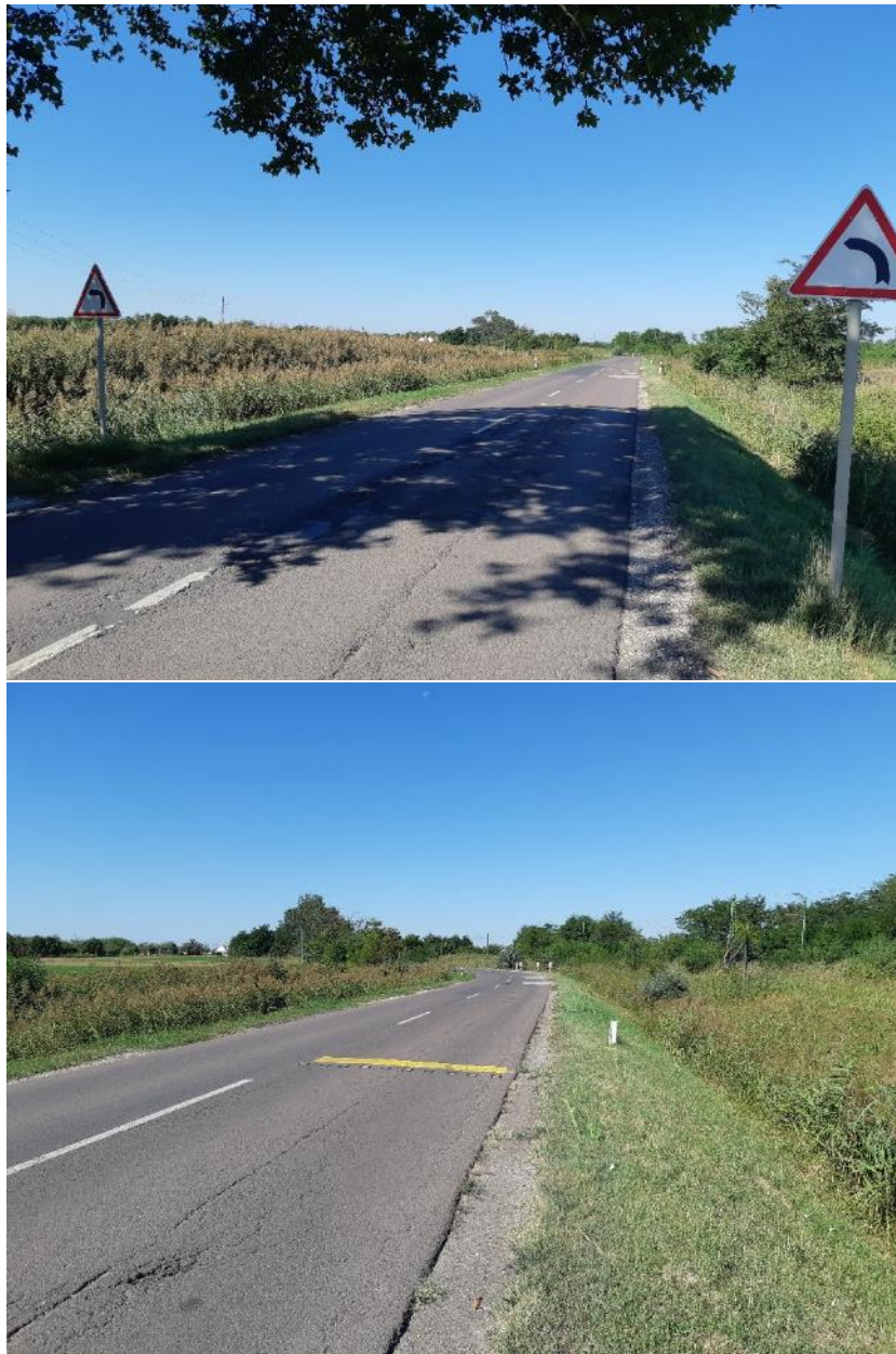
Figure 23: Area of Pilot Action 1 near Cegléd, on road 40 – 1. direction
