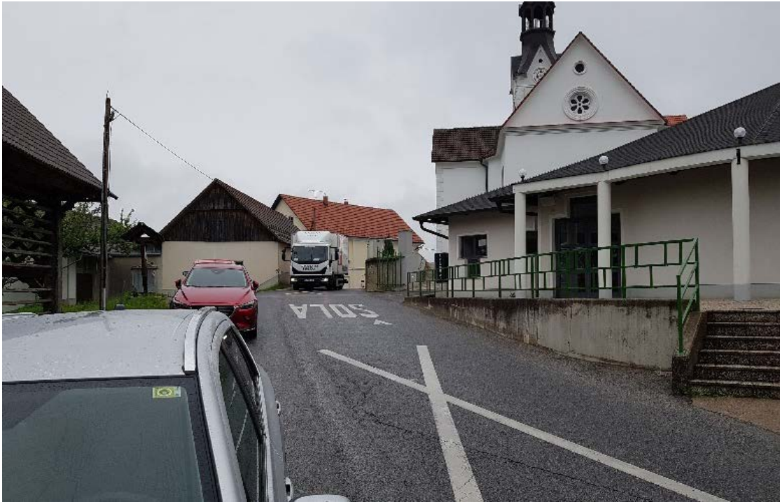
Figure 52 Absence of pedestrian infrastructure on the way to the church and school at Location 2
