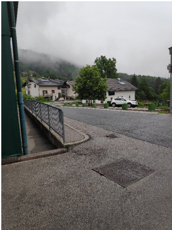
Figure 51 Entrance to the school parking place – poor sight distance on the right-hand side at Location 1
