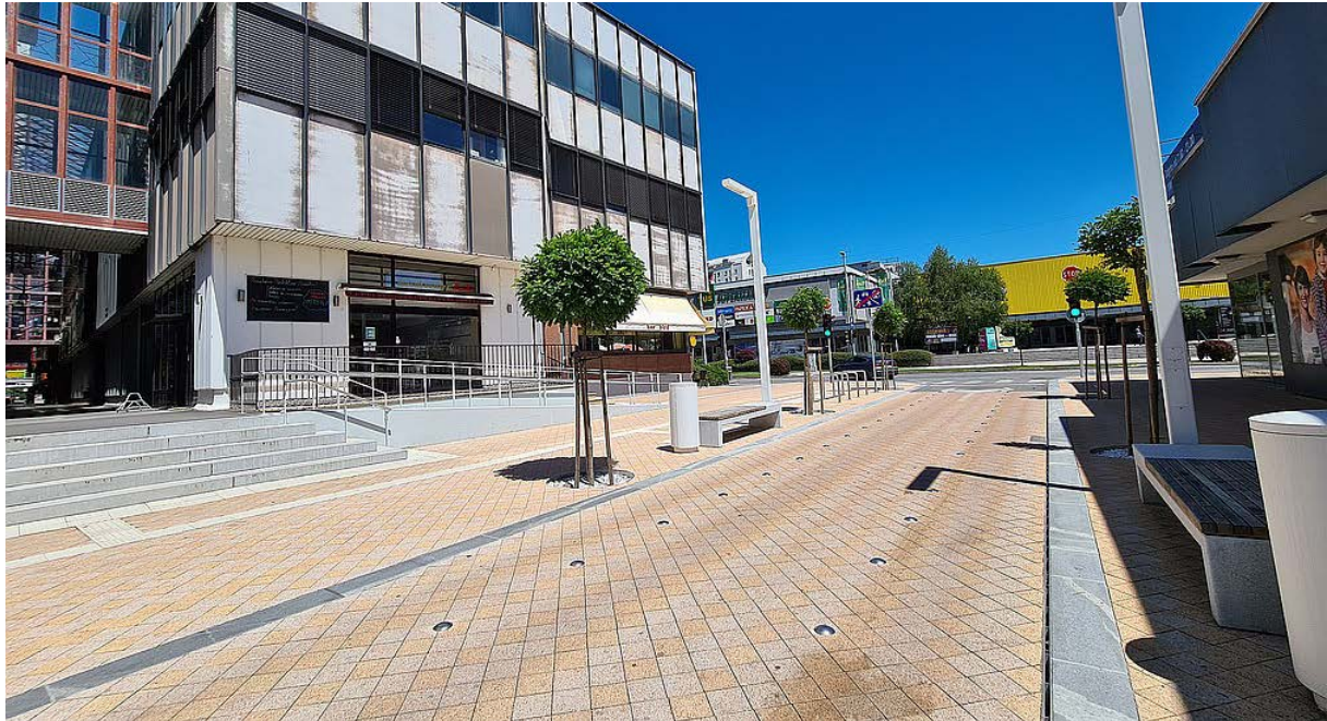
Figure 32 Renovated street and south intersection
