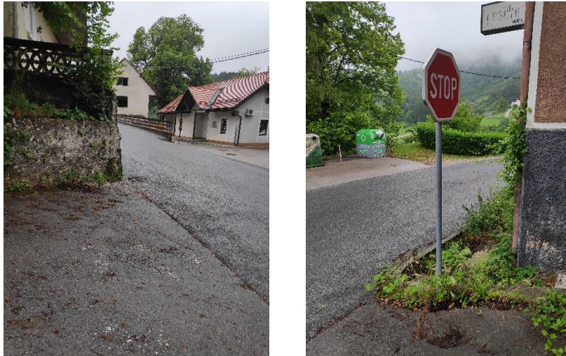
Figure 63: Poor sight distance
