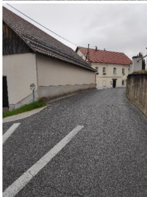
Figure 57 Narrow section of the road in Gabrovka
