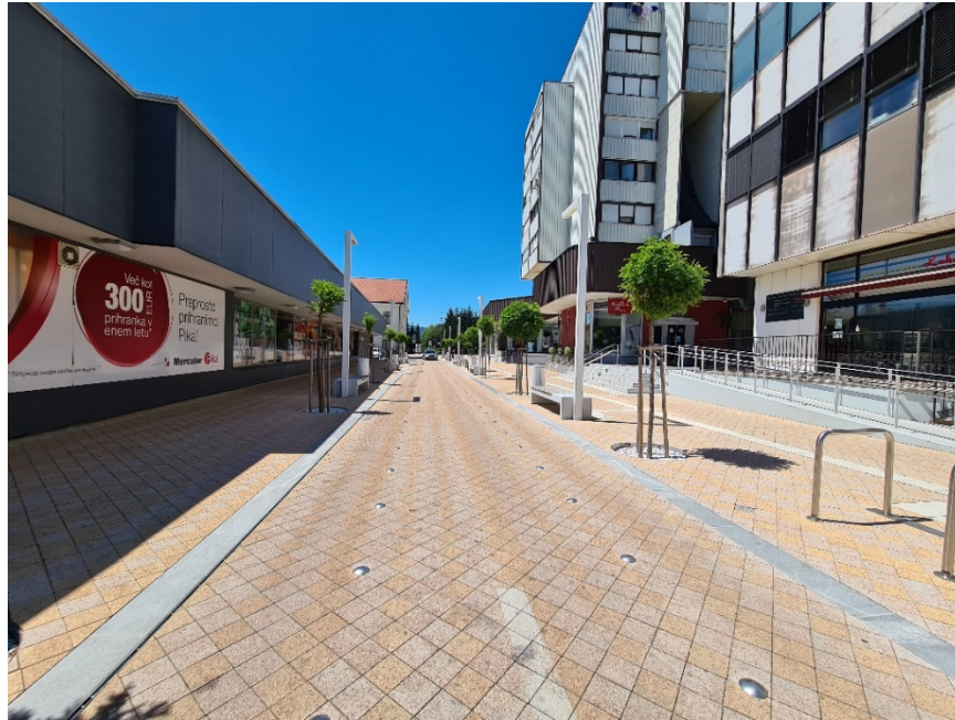
Figure 38: Example of the paving and urban furniture that is proposed to be used in Shared Space in Domžale centre – Kolodvorska cesta
