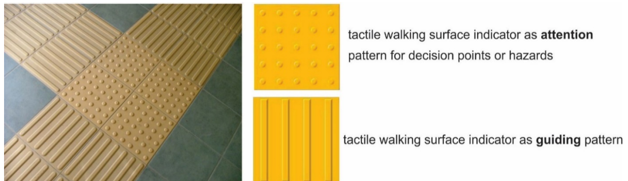
Figure 23 (Two) types of tactile walking surface indicator – attention and guiding pattern
