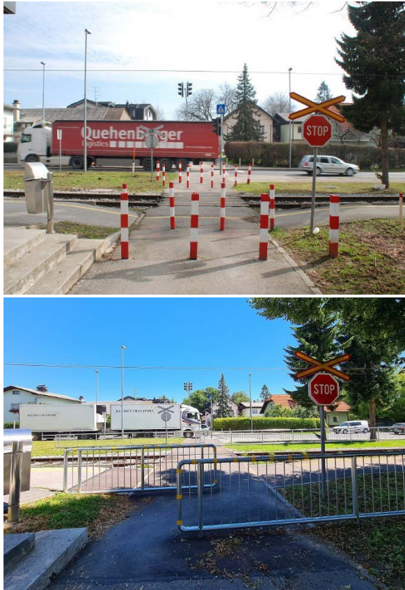
Figure 5 VRU protection at railway crossing before (left) and after (right) 2020 accident
