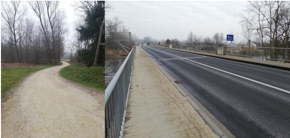
4-5.Figures: Gravel road to Babič Mill at Veržej (left); Mura bridge Petanjci-Radenci (right) Source: Nina Lebar
