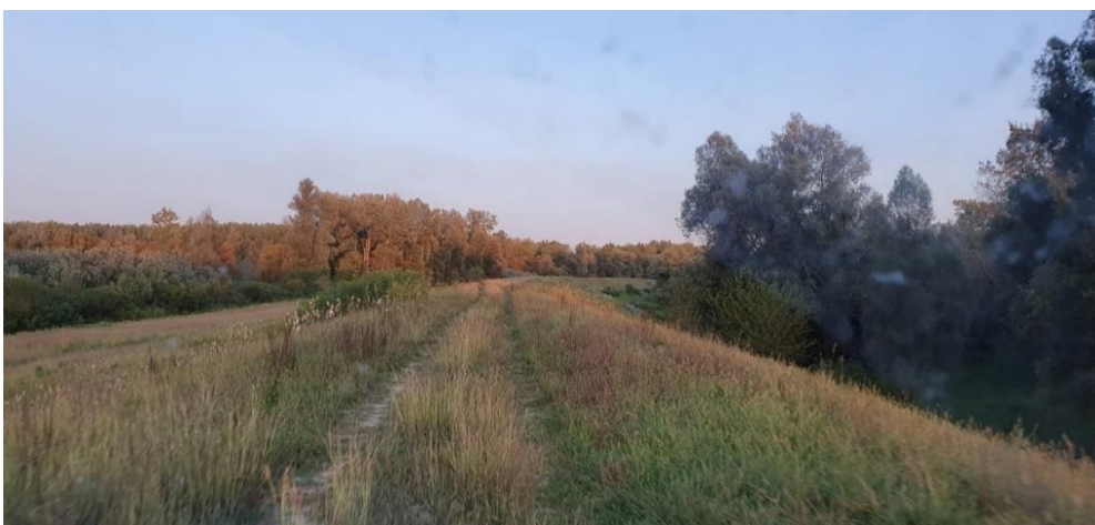
57. Figure: Challenging section on embankment with high grass
