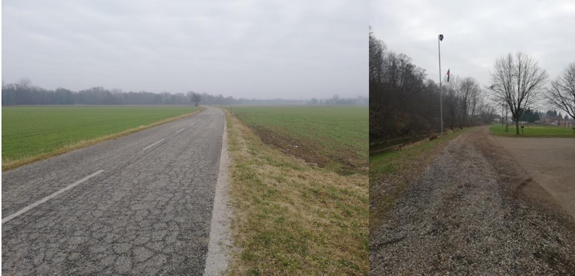
7-8. Figures: Low traffic asphalt road near Razkrižje (left) and unpaved surface between Razkrižje – Šafarsko (right).
