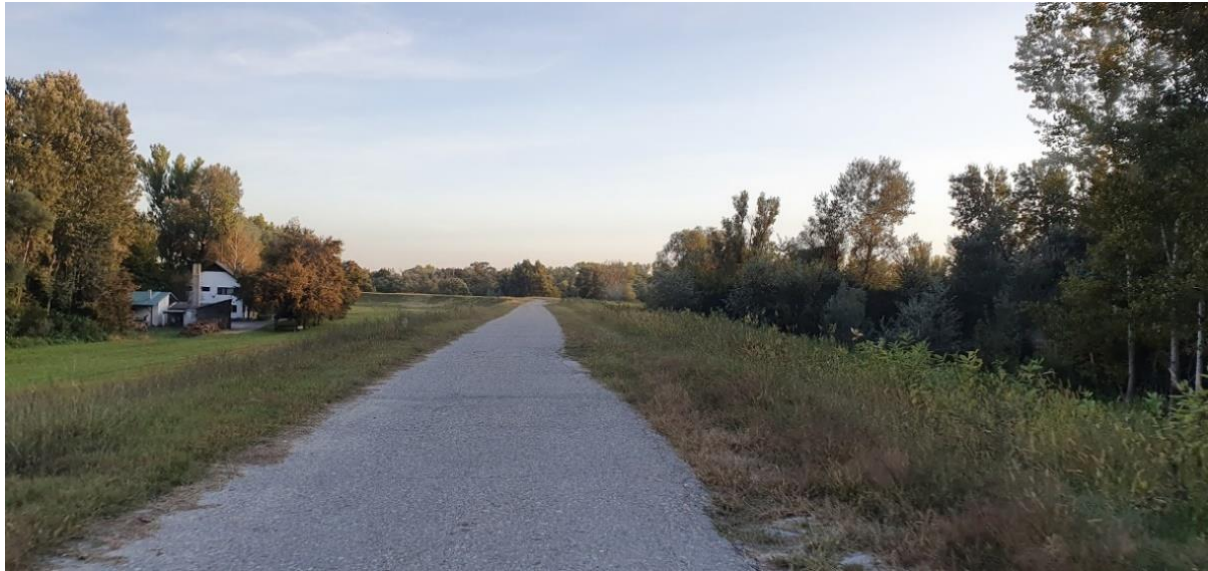
58. Figure: Paved surface o nembankment at hunting house Mesarske livade
