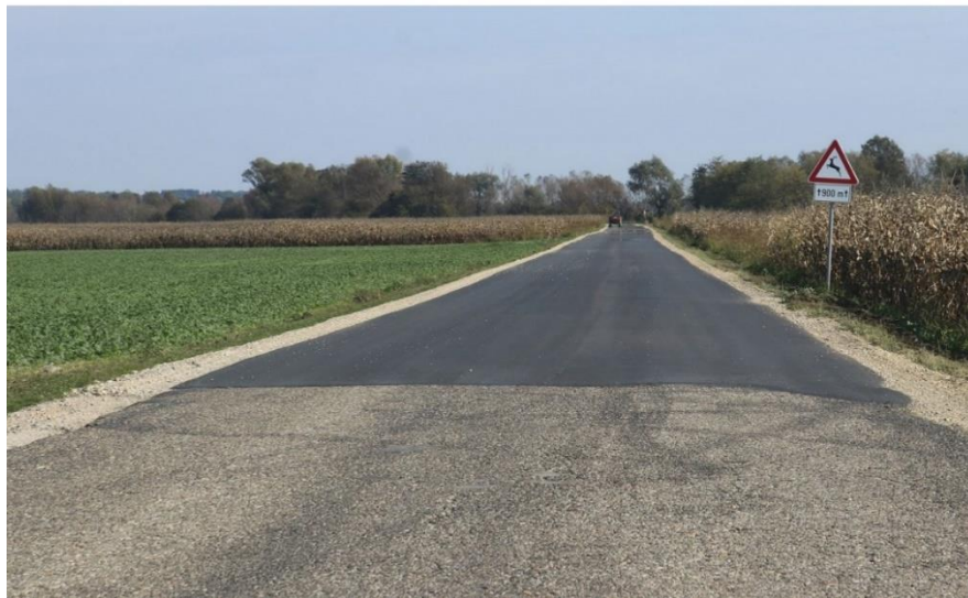
26. Figure: Asphalted road between Đelekovec and Šoderica.
