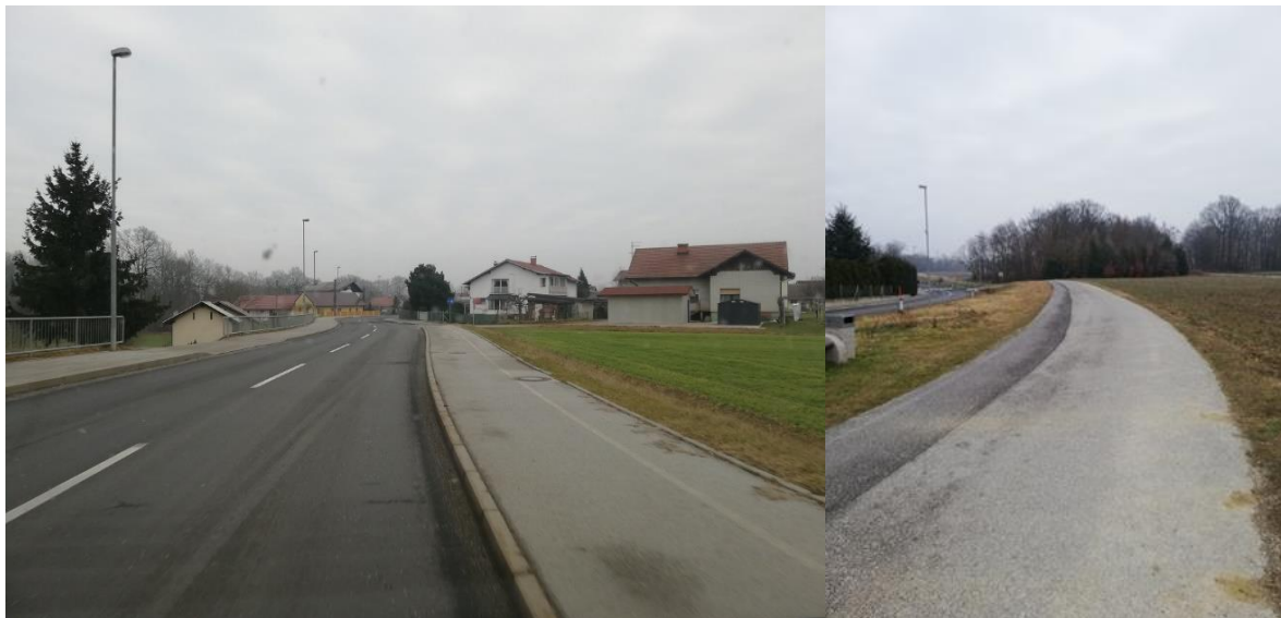
2-3. Figures: Pedestrian/bicycle path inside and seperated path for slow vehicles outside settlements between Radenci- and Vučja Vas
