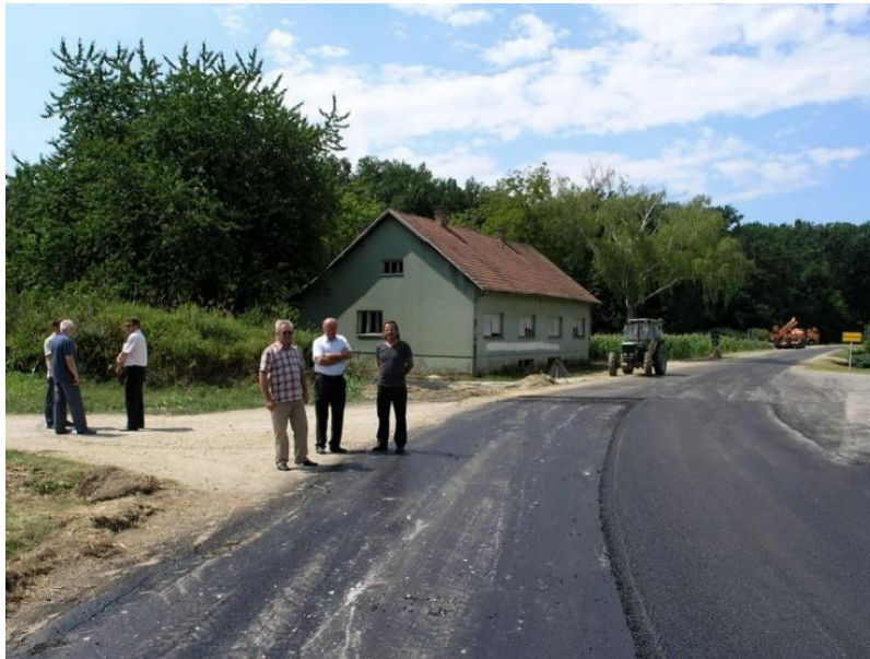
37. Figure: Newly asphalted part of Brodić -Mekiš section
