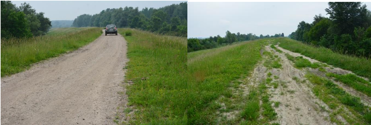
59-60. Figures: Better gravel (left) and dirt/grassy surfaces (right) on embankment in mid-section of the stage
