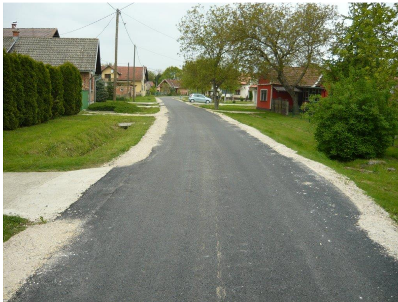
30. Figure: Asphalted road in Sigetec
