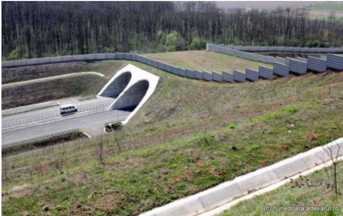
Figure 31. The tunnel. Source: http://www.cnadnr.ro/en/proiecte/proiectare-si-executie-autostrada-lugoj-deva-lot-3 . Report on the environmental impact for the Project: Lugoj-Deva Highway km 0+000-100+014 - http://www.anpm.ro/documents/12220/2231306/RIM+22.11.2016.pdf/c5ea415b-cd85-4dd1-8392-a1219323da2b and https://adevarul.ro/locale/hunedoara/autostrada-lugoj-deva-ecoduct-finalizat-7_5ca76644445219c57e240f86/2_5ca76699445219c57e241813.html#photo-head
