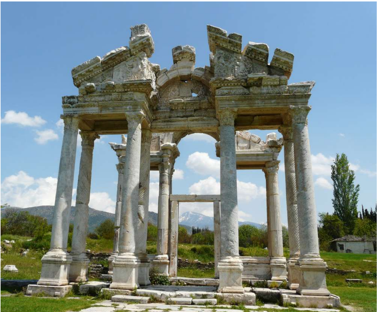
Figure 4.4. Aphrodisias (Turkey), tetrapylon reassembled by anastylosis (photo Zigomar, https://commons.wikimedia.org/wiki/File:Aphrodisias_tetrapylon_2009_04_27.jpg ).
