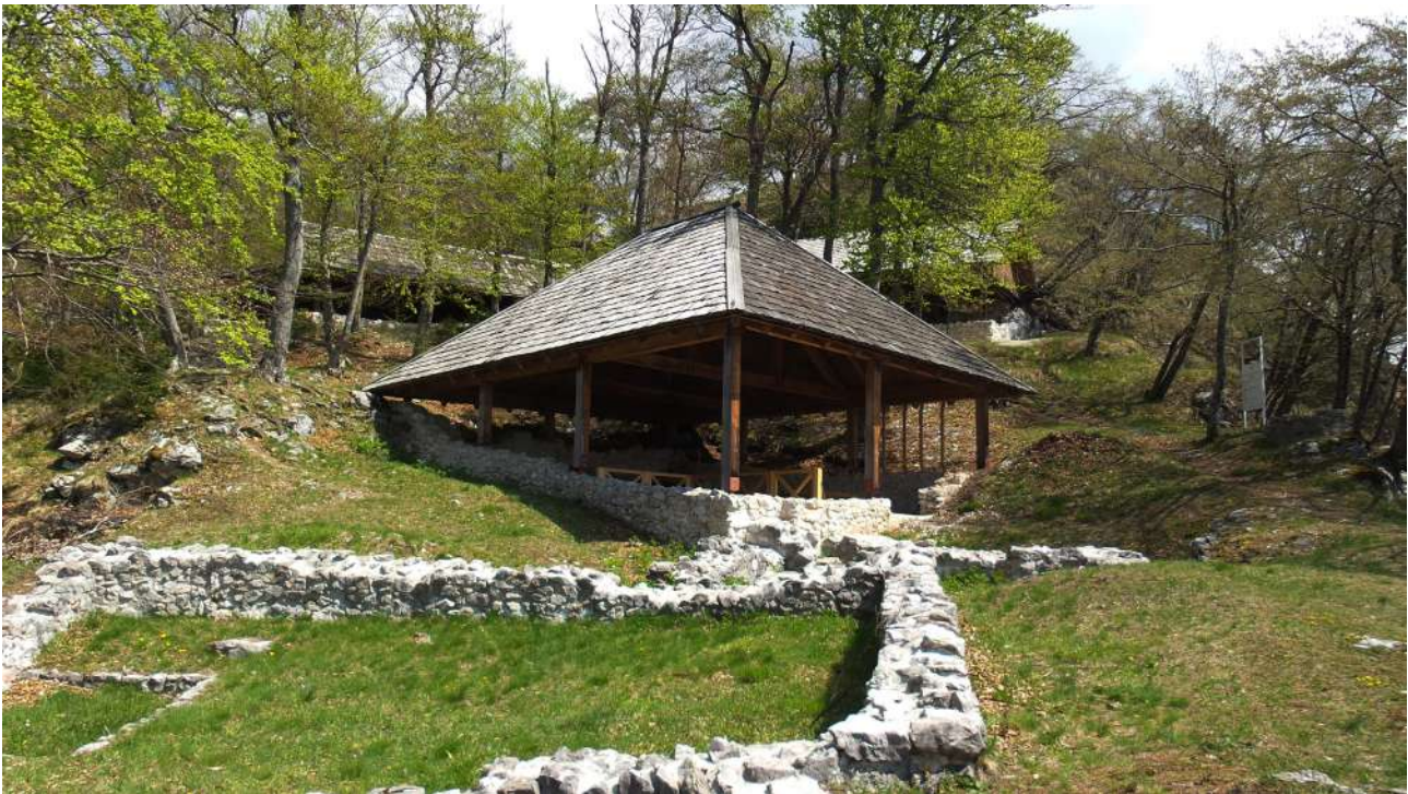
Figure 4.8. Ajdna nad Potoki (Slovenia), wooden shelters above the remains of the late antiquity hilltop settlement (photo Katharina Zanier).
