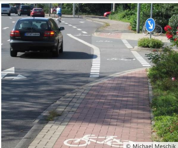
Figure 23: Cycle track next to the lane for the motorists at an intersection
