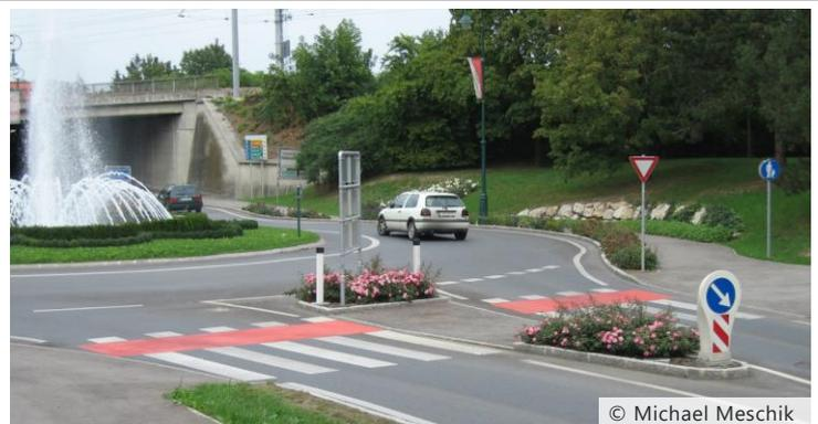
Figure 26: Segregated track around the roundabout
