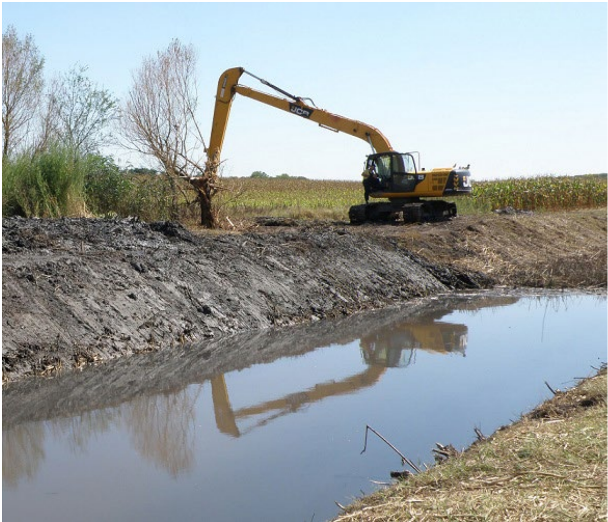
Figure 14: Dredging of the ameliorative canal. The grass strips of canal banks are permanently covered by silt, creating an open surface rich in nutritive materials.
