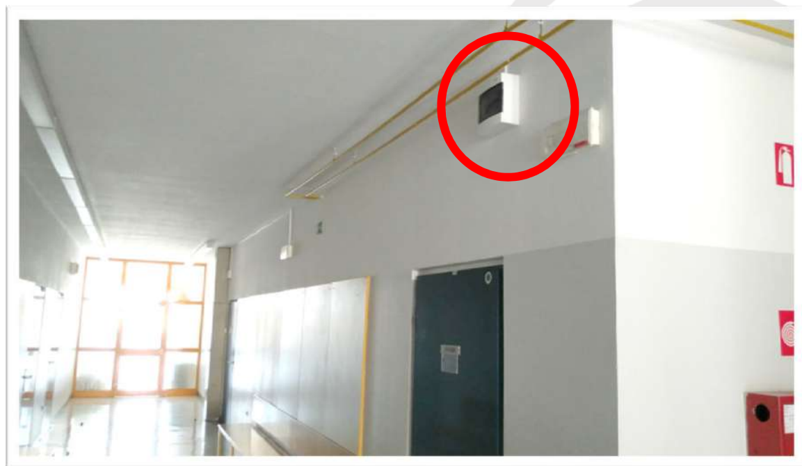
Gateway in the first floor hallway
