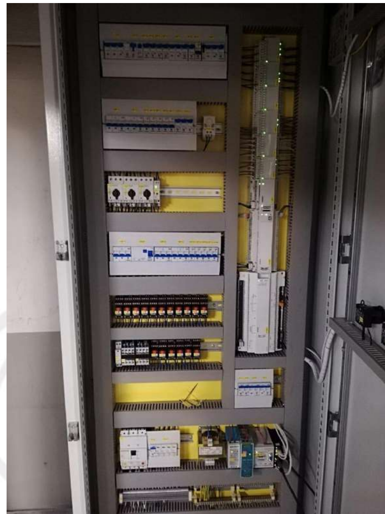
Control cabinet for Heating Station
