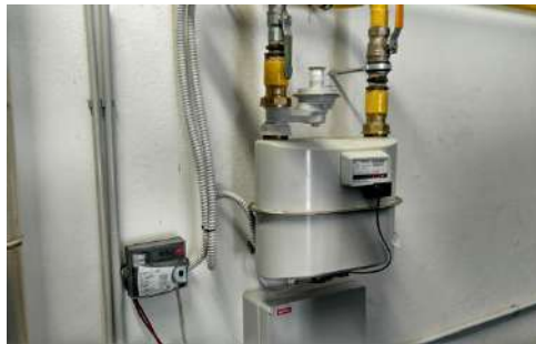
Gas counter and calorimeter
