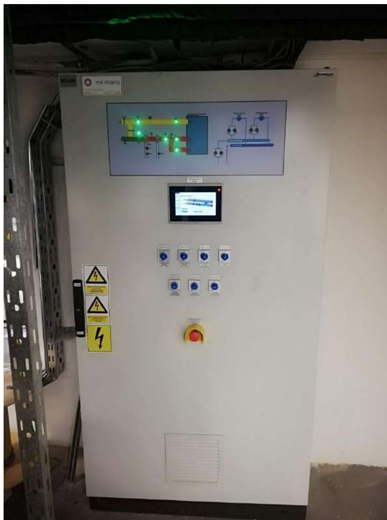
Control cabinet for AHU and Cooling Station (Water Chillers and pumps)
