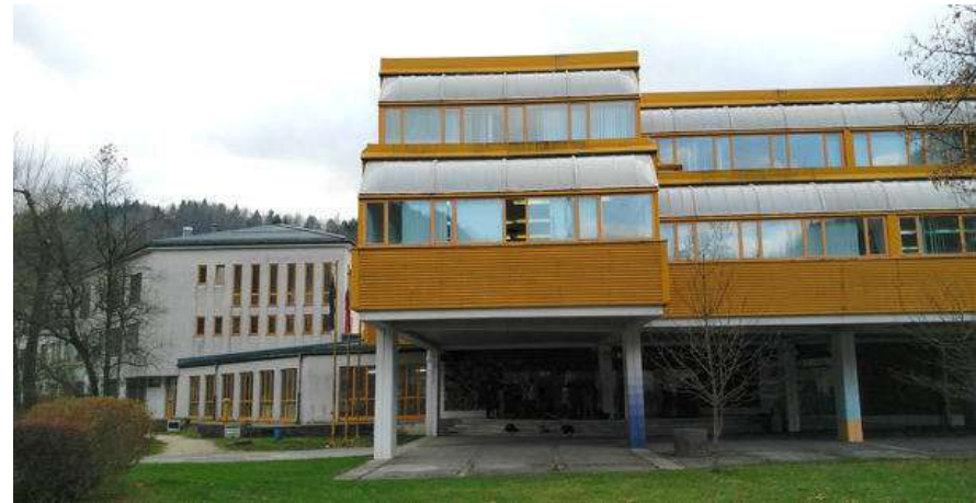
Some classrooms are very exposed
