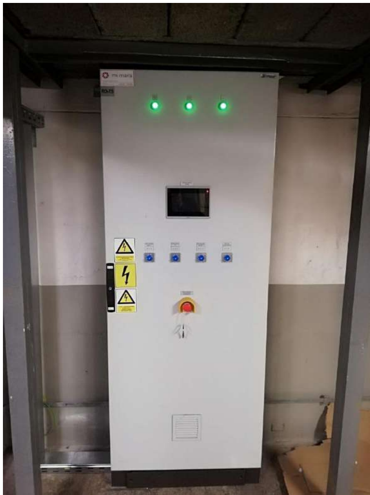
Control cabinet for Heating Station
