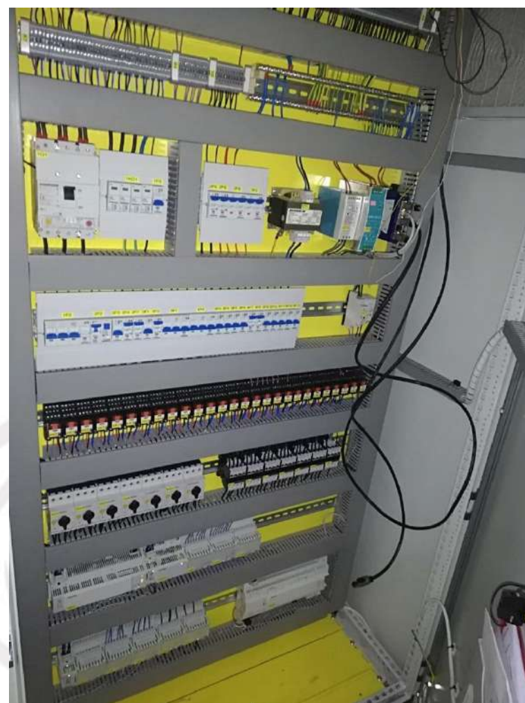
Control cabinet for AHU and Cooling Station (Water Chillers and pumps)
