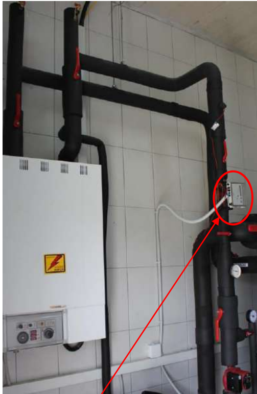
Calorimeter for electric boiler Siemens UH50-A45C-BA06-E
