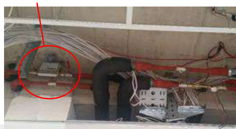
calorimeters on ground floor
