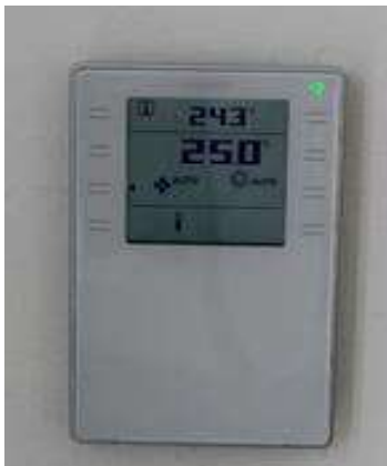
Room operator unit SIEMENS QMX3.P34
