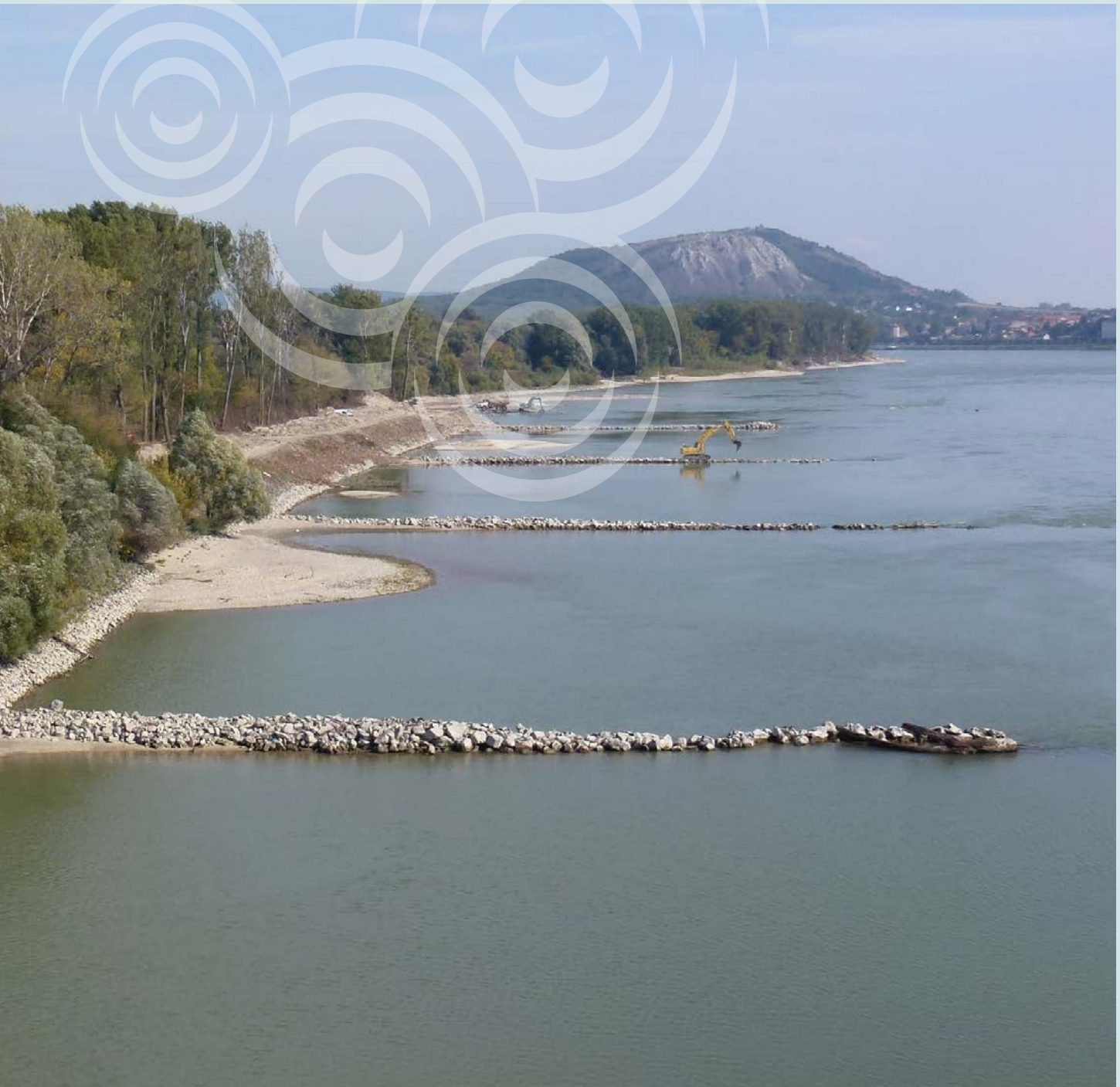
Optimisation of river engineering structures to reduce erosion (© IWA/BOKU)
