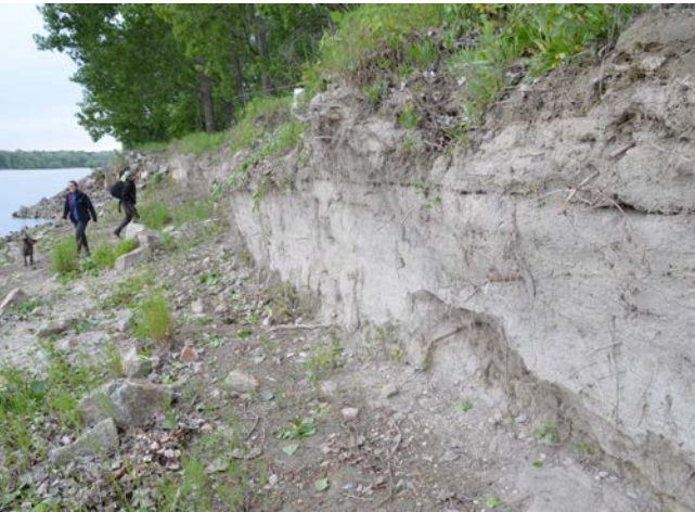
Figure 27: Removal of bank protection at the Slovakian Danube (© WRI)
