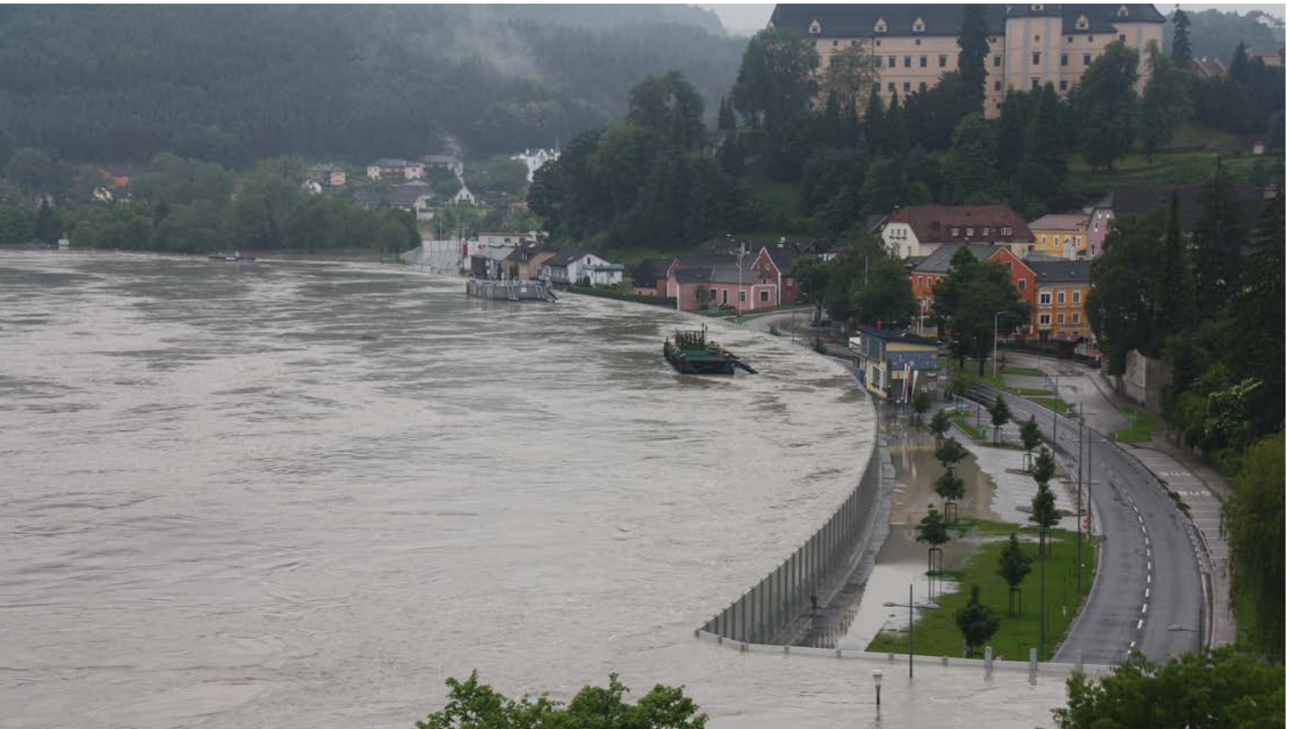
Figure 4: Mobile flood protection Danube River, Austria (© Robert Zinterhof)
