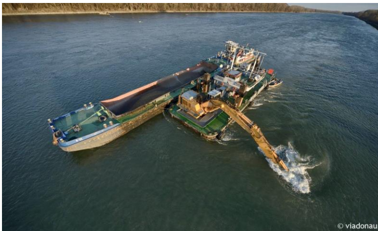
Figure 3: Dredging in the fairway.
