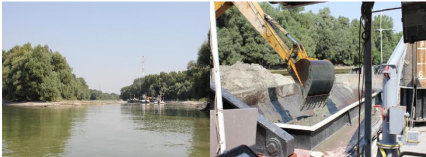
Figure 6 Dredging activities for side-arm reconnection in Hungary
