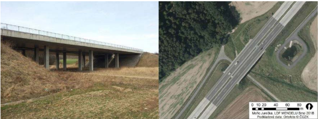
Fig. 33: Locality 2: Underpass Bílov.
