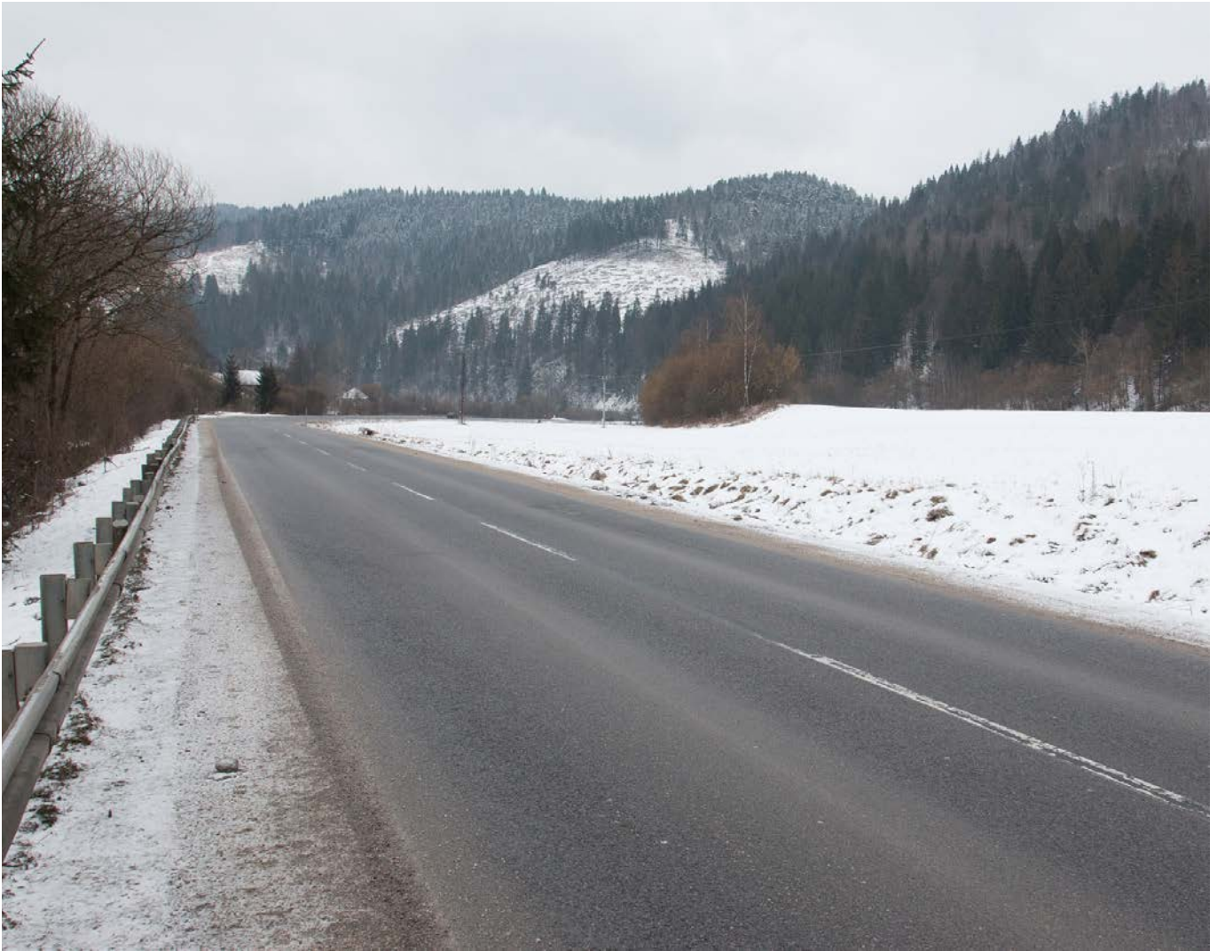
Fig. 33: View of the corridor zone intersected by the 2 nd class road II/520. Note that forests approach the road on both sides of the road, which is very suitable for wildlife movements.
