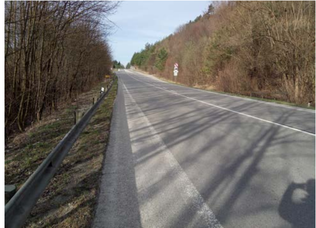
Fig. 58: Photo of the corridor and the 1 st class road I/61. Dense vegetation approaches the road from both sides, which is preferred by wildlife for road crossing.
