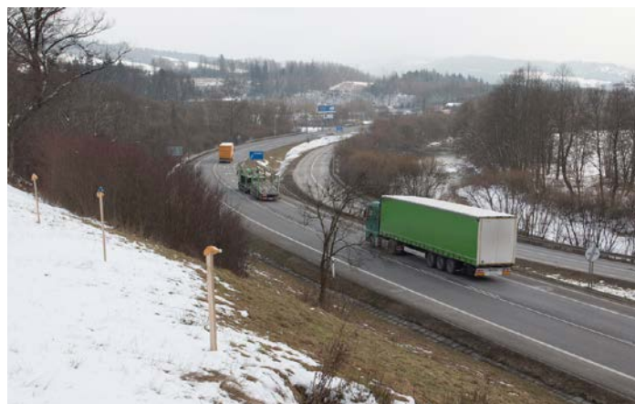
Fig. 30: View of the corridor zone and 1 st class road I/11 and II/11B. Note: the river flows parallel to the road, posing a serious barrier for wildlife movement.
