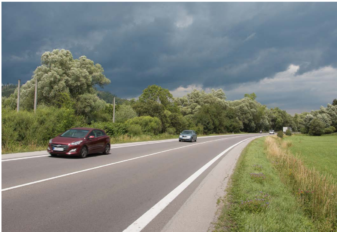
Fig. 39: View of the corridor Povina and the 1 st class road I/11.
