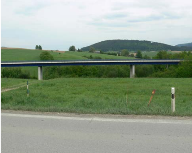
Fig. 8: Middle section of corridor in Jablunkov.
