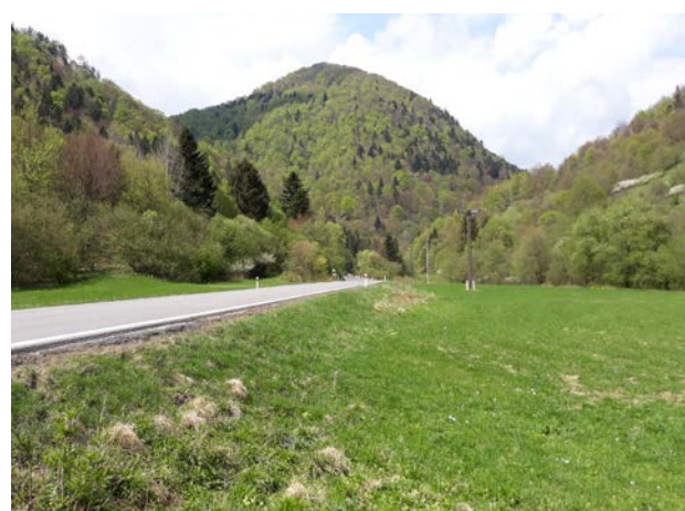
Fig. 50: View of the corridor Sokol and the 2 nd class road II/583. The area is densely forested and facilitates frequent wildlife movement.
