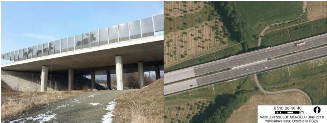
Fig. 41: Locality 10: Underpass Jezernice.
