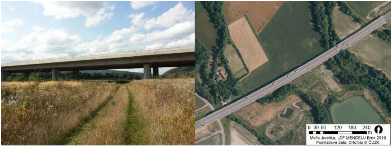
Fig. 43: Locality 12: Landscape bridge Odry.
