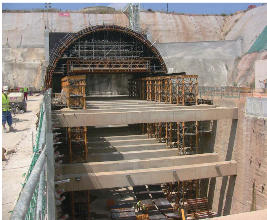
Fig. 63. Tunel cut-and-cover, Extindere cale ferată, Terrassa, Spain (Foto Ulma Construction 1) )
