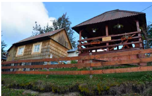
Fig 21: In forested karst areas wood has traditionally been the major material for construction and is again becoming more popular (Apušeni NP, photo A. Golob).
