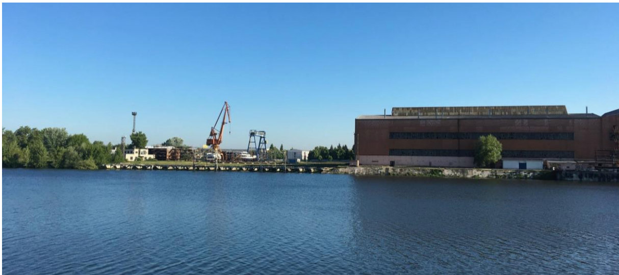
Fig. 37: The view of the hall buildings and the new lift ship in Komárno from 2017 (source: foto/archive by Martin Dubiny).
