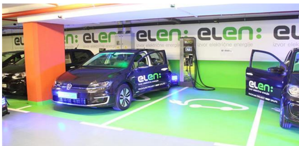
Figure 18: Charging station for E-cars
