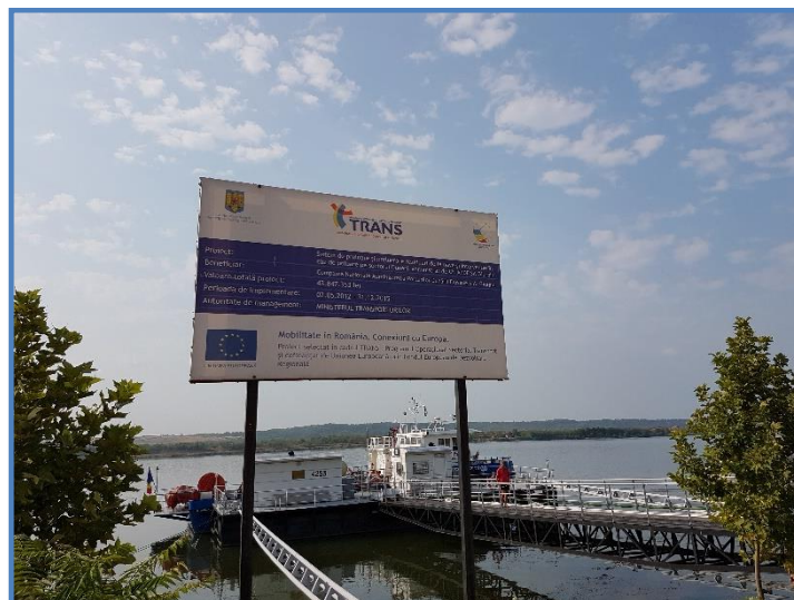
Figure 44 Residues receiving system in the Port of Drobeta Turnu-Severin
