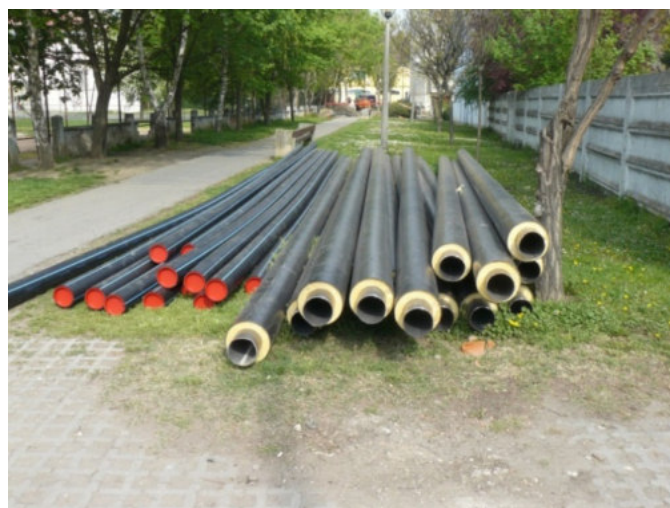
Figure 2: Pipeline with uninsulated plastic and insulated steel utility pipe
