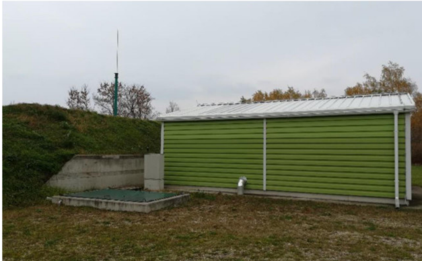
Figure 19: (Re)injection well Le-3g with engine house
