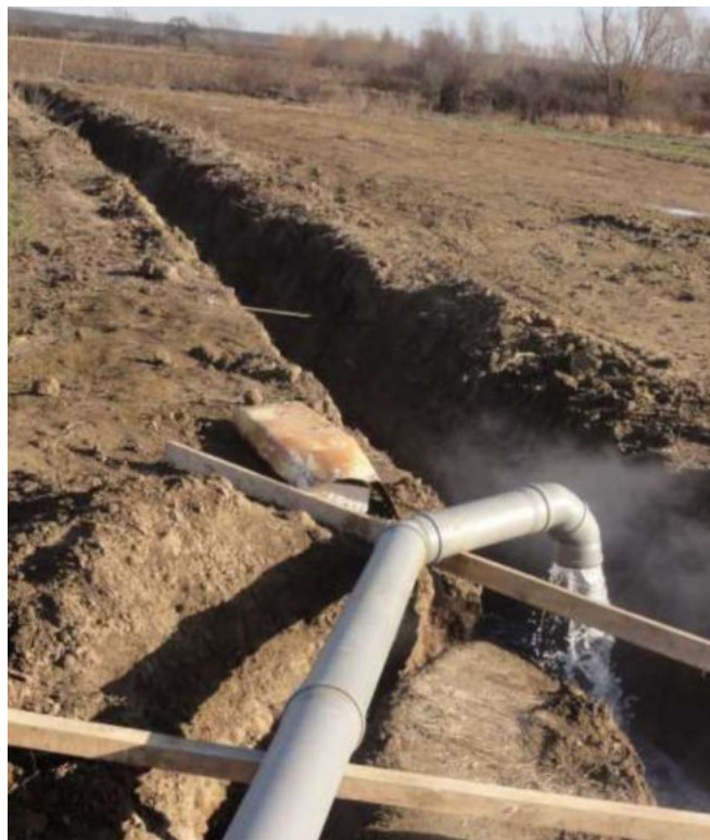
Fig. 7: The discharge of the cooled geothermal water at the vicinity of the well (Photo: T. Bilić)
