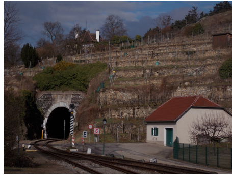
fig. 20: railway-tunnel Dürnstein. source: Isidora Kisin, U-NS
