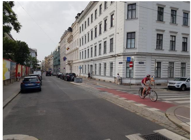
Figure 40. Vienna, Austria, example of a cycle track without obligation. Cyclists may prefer to use the carriageway downhill in its direction and uphill to use the track as the only legal possibility in this street. Such special application of a cycle track is marked with a different horizontal and vertical sign, see chapter 10.1. Source: Sindikat biciklista
