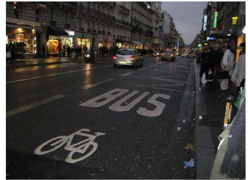
Figure 134. Shared bus-bike lane in Paris, France. Source: A Summary of Design, Policies and Operational Characteristics for Shared Bicycle/Bus Lanes, 2012). [1]
