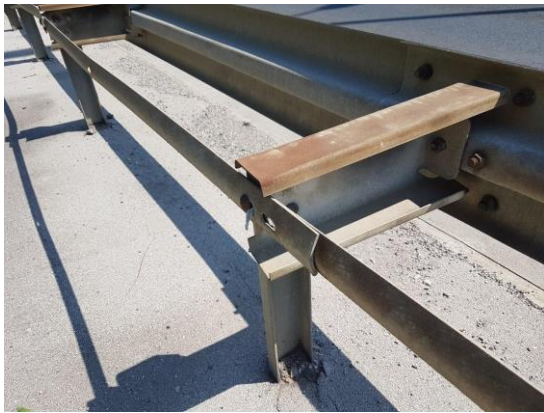
Figure 37. Example from Croatia: parapet between cycle track and motorway with the inner side trying to protect cyclists from injury – almost good but still with a short sharp edge. Source: Sindikat biciklista
