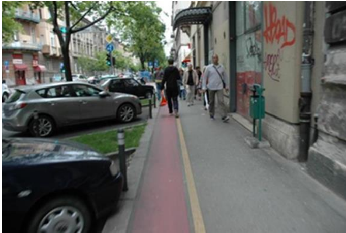
Figure 28. Bad example of a cycle and pedestrian track from Croatia. Source: Sindikat biciklista
