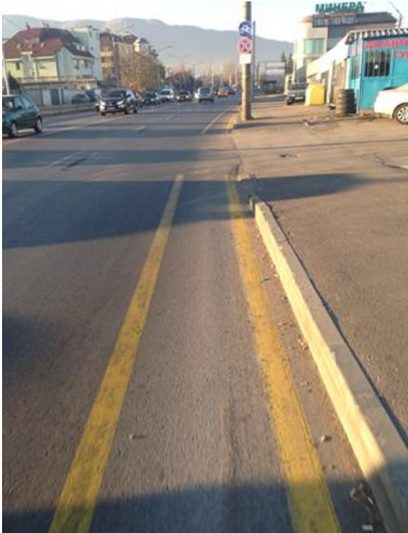
Figure 14. Example of bad cycle lane from Bulgaria. Source: DCP design standards
