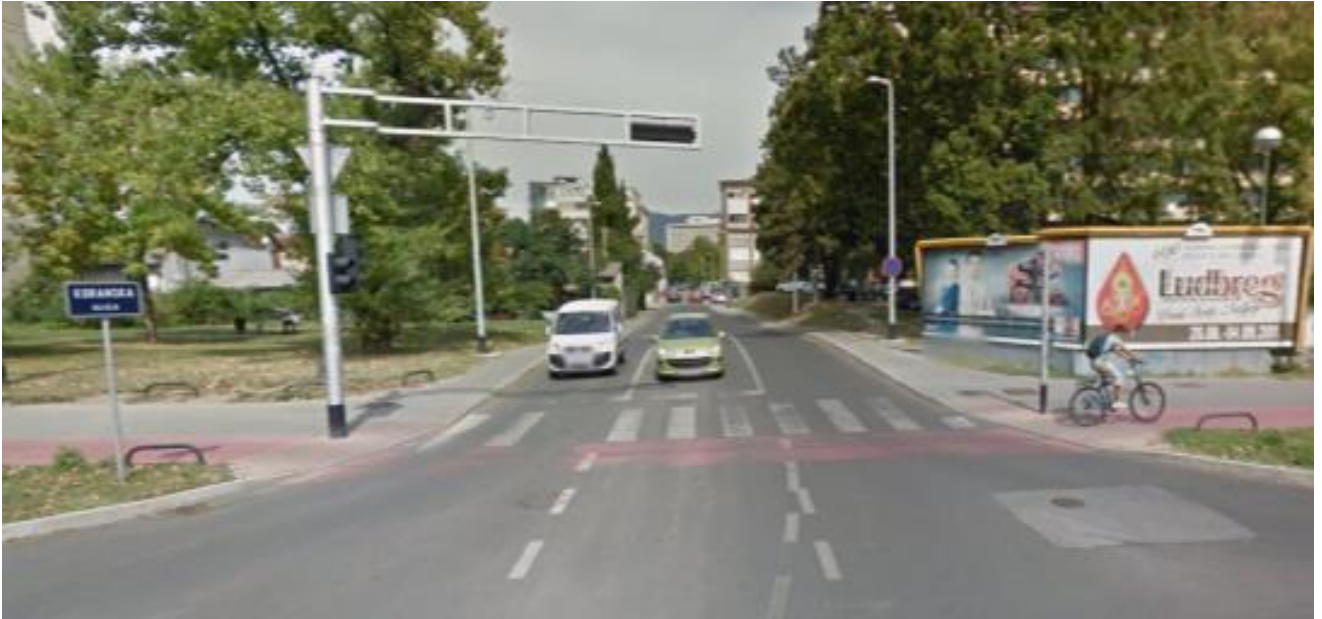
Figure 126. Zagreb, Croatia: faded signalization of a cycle track crossing an intersection. Right turning cars from the priority road are not aware of cyclists having advantage. Source: Sindikat biciklista
