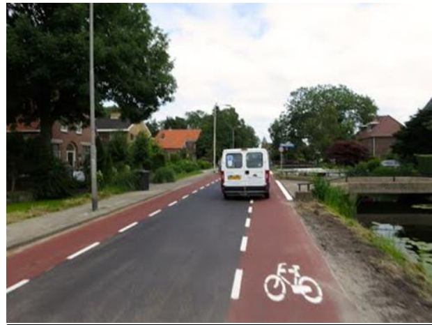
Figure 18. Example of advisory cycle lane from Netherlands. Source: PSU Delft multimodal transportation 2013
