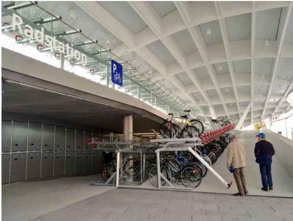
Figure 92. Bicycle parking facility with lockers at Salzburg Central station. Source: Andreas Lindinger
