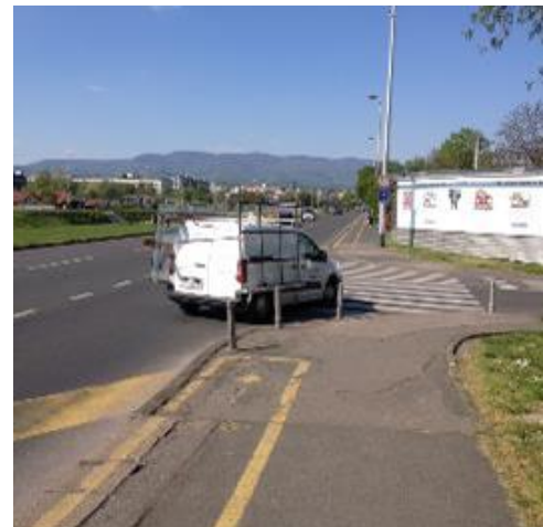
Figure 47. Zagreb, Croatia, a cycle track along the 6-lanes city avenue ends before a junction of a minor non-priority street and starts again after the intersection. Source: Sindikat biciklista
