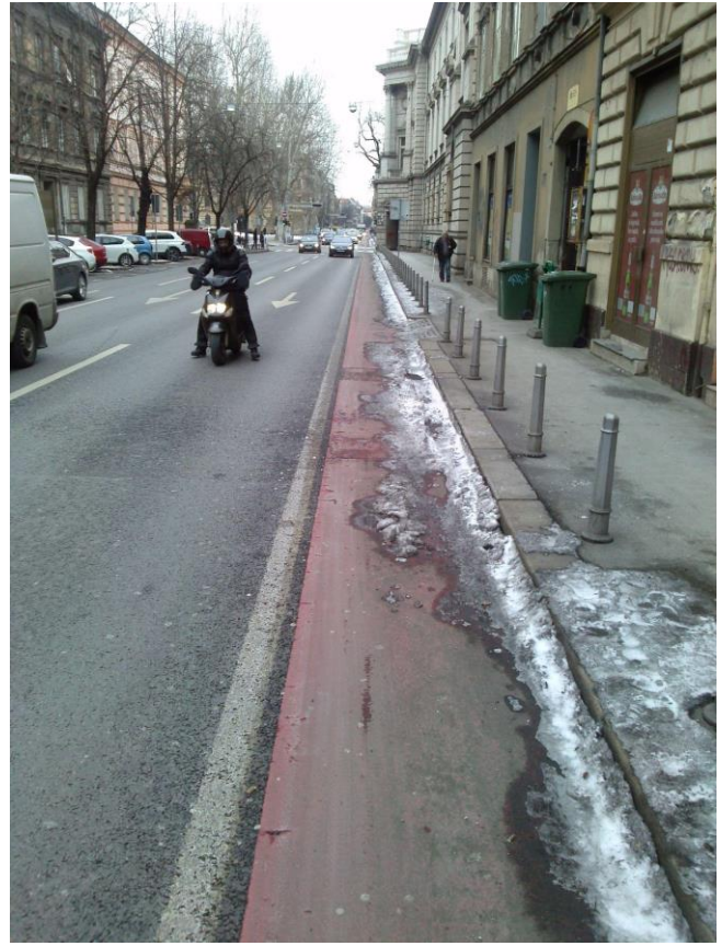
Figure 131. Example of poorly maintained cycling infrastructure in winter conditions. Source: Sindikat biciklista
