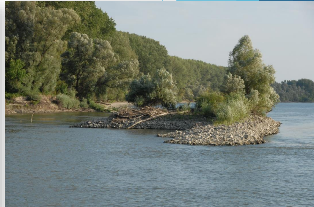
Disconnected T-Groyne in Danube for water way transport to stabilize fairway (Wolfgang Kraier).
