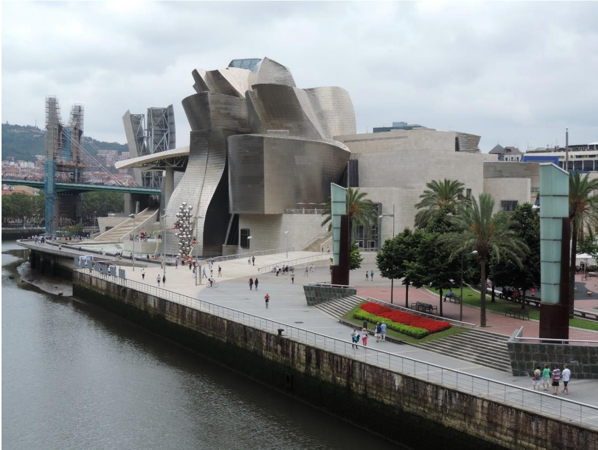
The Guggenheim Museum, Bilbao Photo by Tamara Rátz
