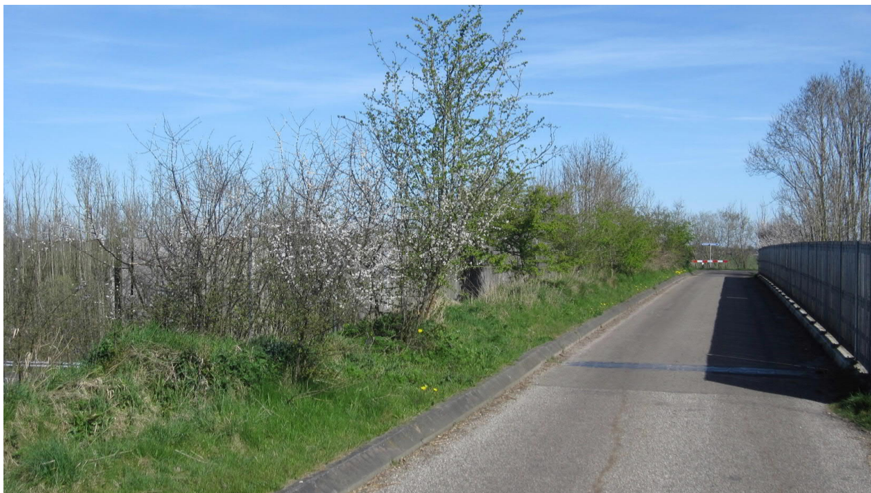
Adapted existing local viaduct
