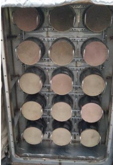
SCR at installation
