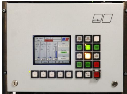
Local Operator Panel (LOP), customer interface
