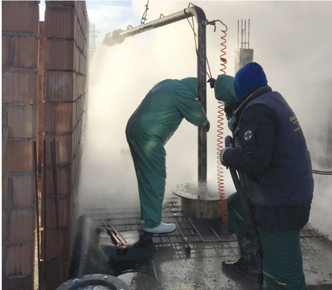
Construction and testing of new production well BB-1
