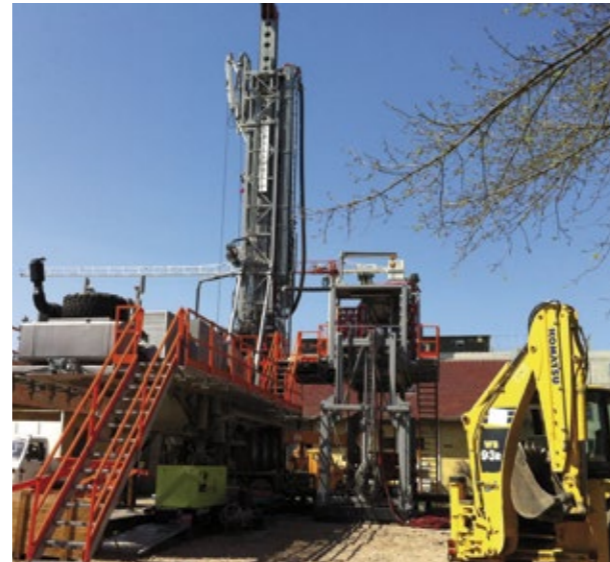
Drilling rig at work in Szeged
