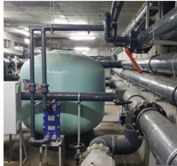
Completed subsurface installations of the aqua park
