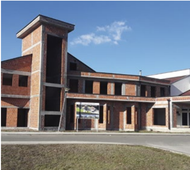
Domaljevac Spa – under construction (November, 2018)
