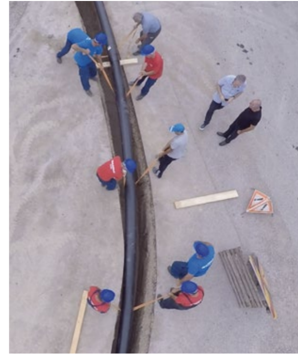
Construction work of the geothermal heating system
