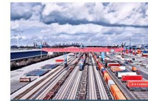
Intermodal Rail Terminals
