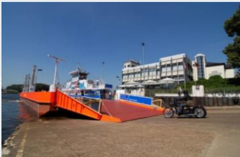
Diesel Electrical Car Ferry with Battery
