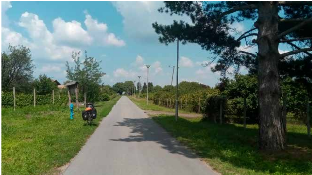
Croatian part of daily section 46 (from Hungarian border to Grabovac/Sokolovac) already meets the Essential and Important criteria in terms of route infrastructure.
