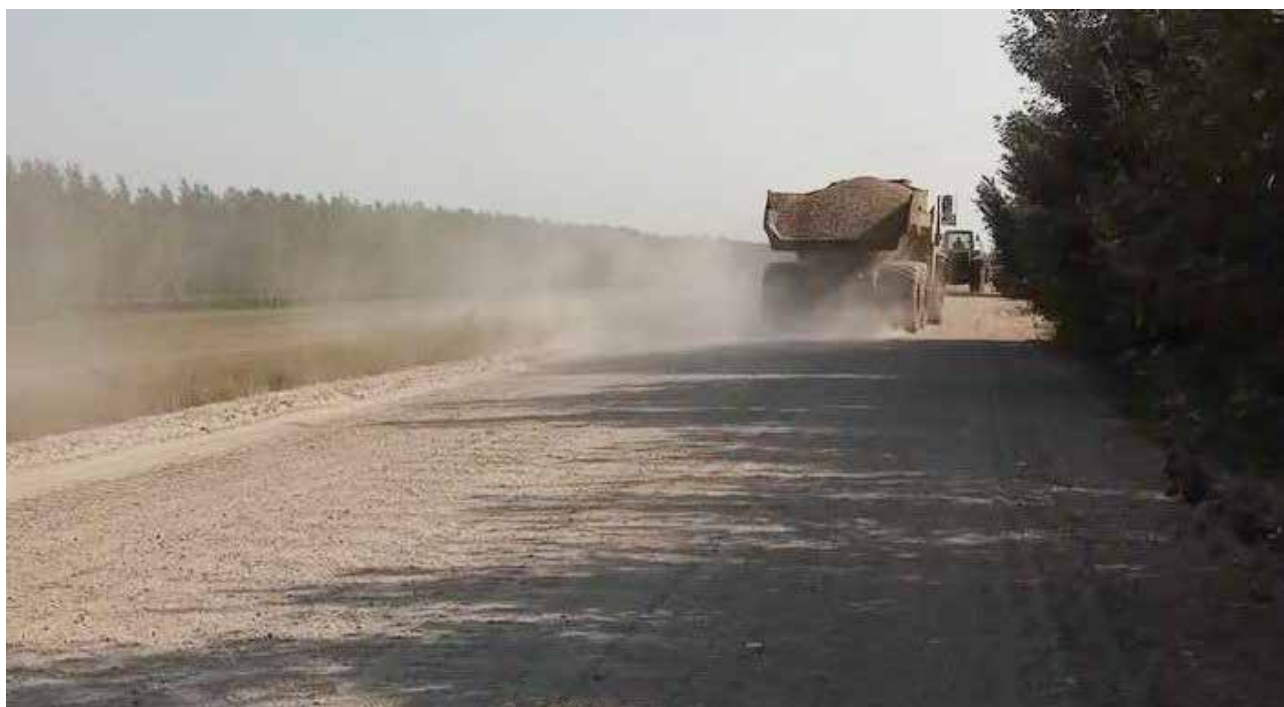
Gravel surface on roads shared with motorised traffic can also create environmental challenges. Photo from section 61: Kovin - Stara Palanka / Bela Crvka
