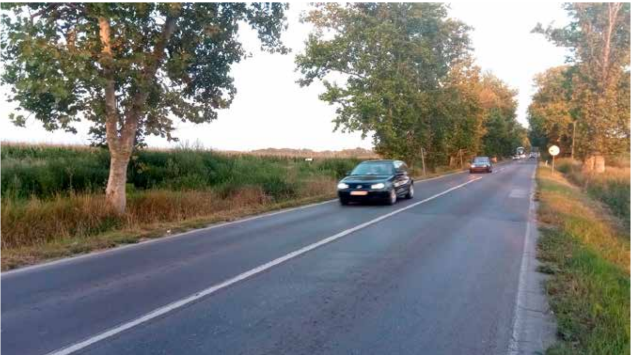
Public road with high traffic and no cycle facilities between Zemun and Belgrade.
